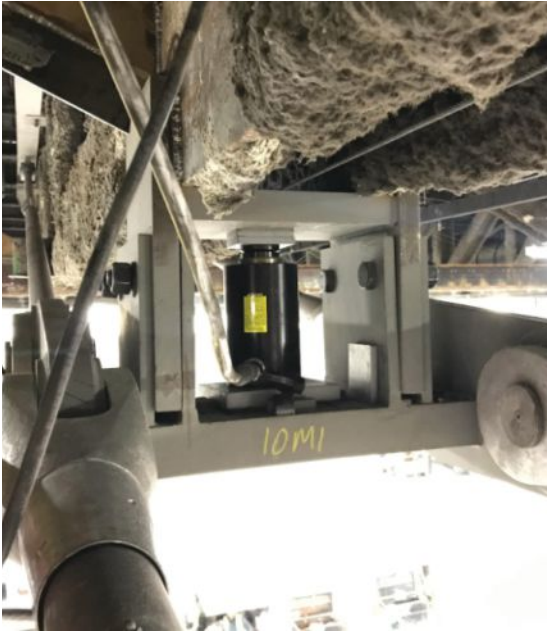
above: A hydraulic jack was used at external post-tensioned bottom chord queen post locations.
