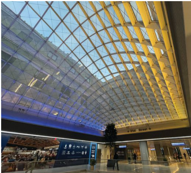
above, left, and below: The peaks of the steel-framed arched skylights in the main concourse rise to a lofty 92 ft above the floor.
