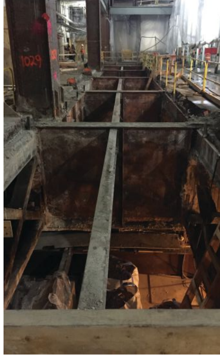
left: The selected design scheme reused three existing 150-ft-long steel trusses.
