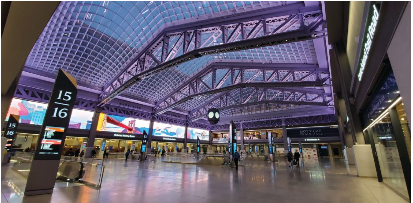
above, left, and below: The peaks of the steel-framed arched skylights in the main concourse rise to a lofty 92 ft above the floor.
