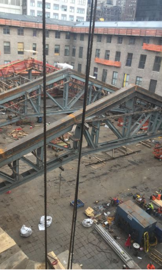
left: The selected design scheme reused three existing 150-ft-long steel trusses.
