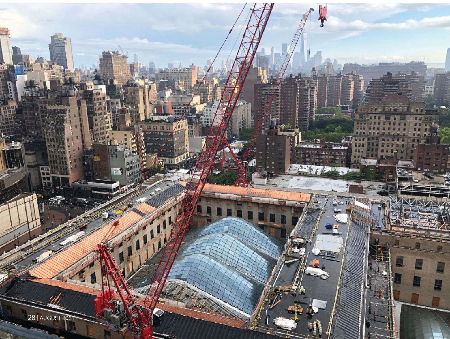
below: Installing the skylights.
