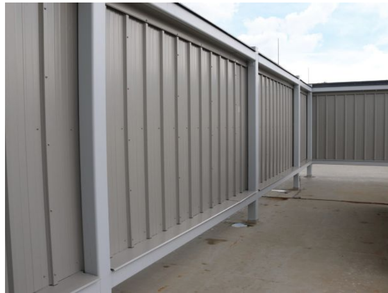
above and left: The steel-framed roof screen is wrapped in the same metal panel system as the rest of the building.
