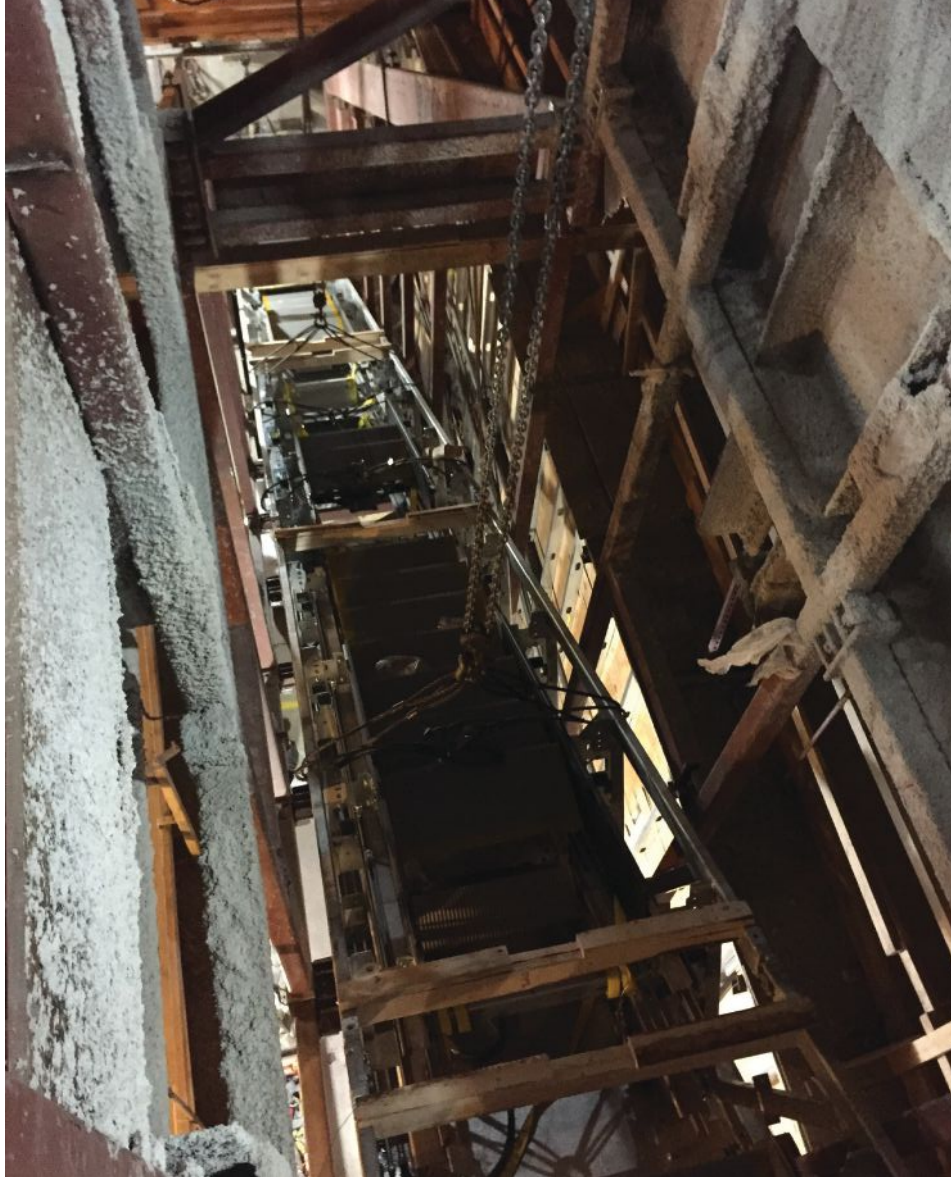
above: A view of the escalator rigging through a finished opening.
