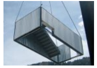
Preinstalled stairs, embeds and connections improve safety and accelerate the schedule.
