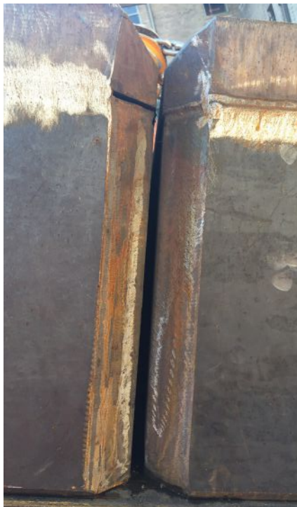
below: Box beam welds.
