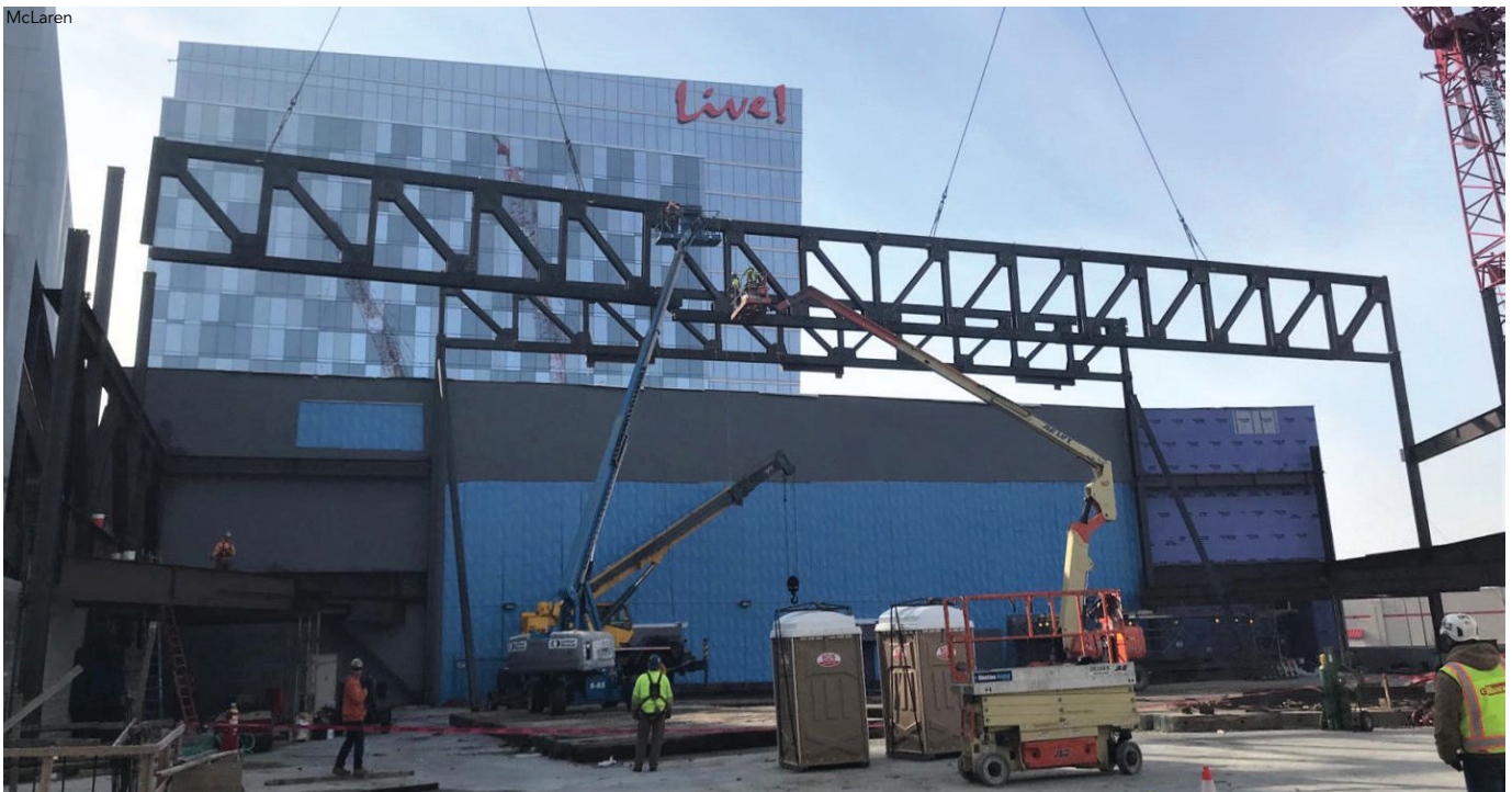
above: Erection of a 174-ft-long truss that supports the suspended seating tiers.
