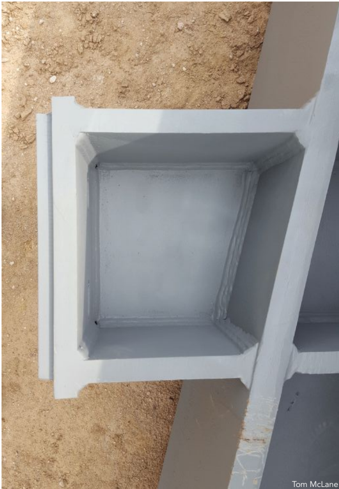
left: Steel framing above a bearing pad prior to installation.
