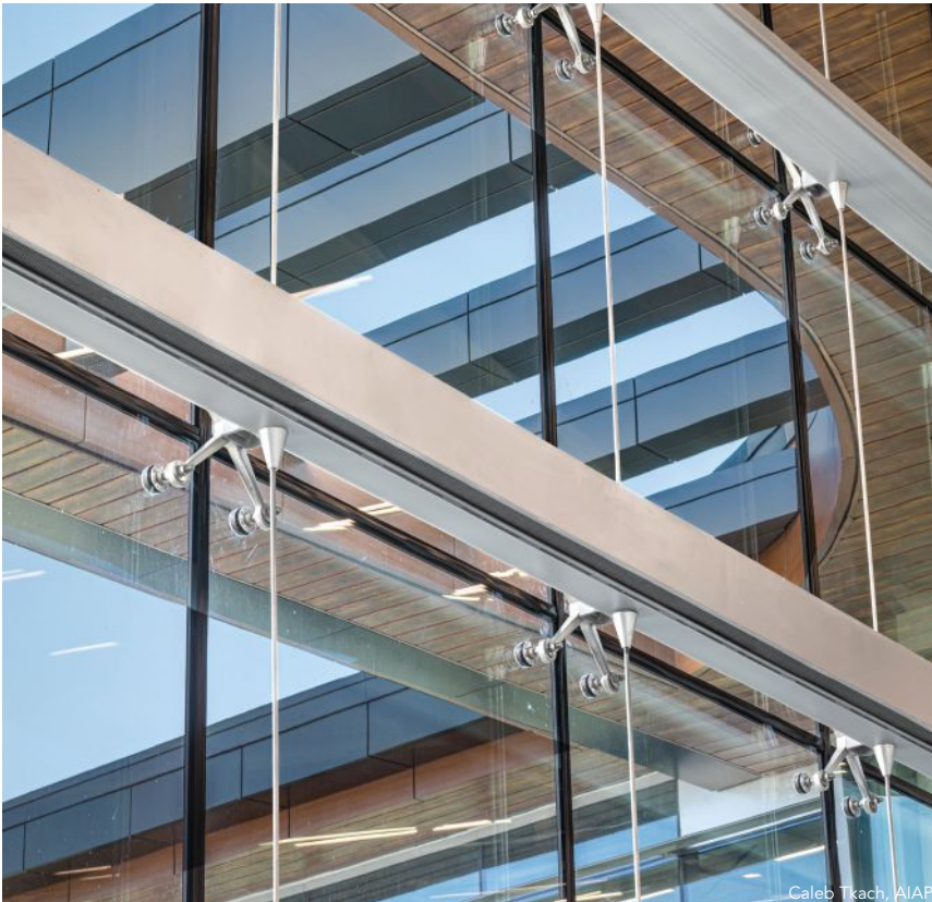
left: The point-supported glass around the curved atrium façade added significant point loads to the roof framing due to the tension in the wall system's vertical cables, thus requiring considerable coordination between the various team members.
