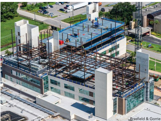
Steel framing being installed on the existing building.
