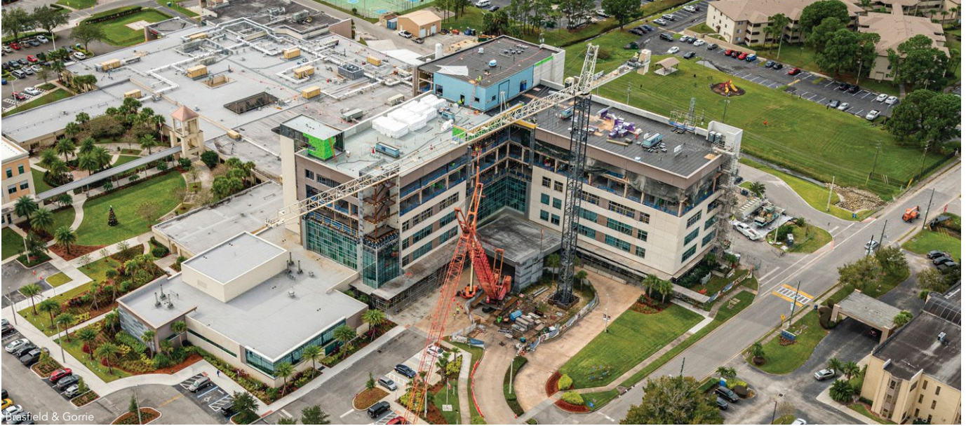
above: The addition uses 533 tons of steel in all.
