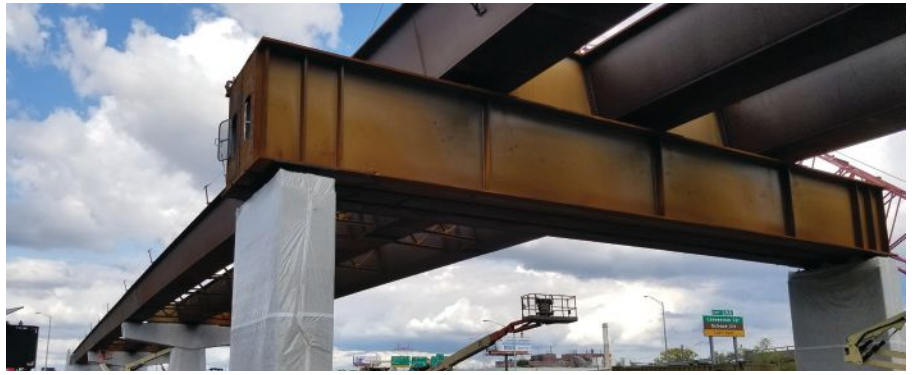
Fig. 11. Completed erection of the framing.
