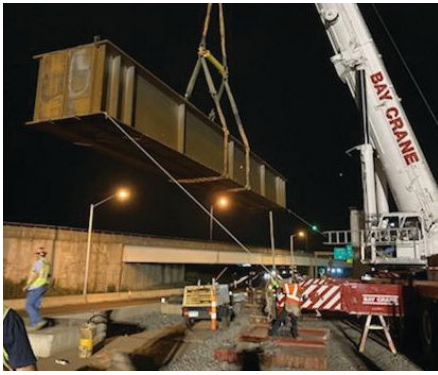
Fig. 10. Erection of the cap.
