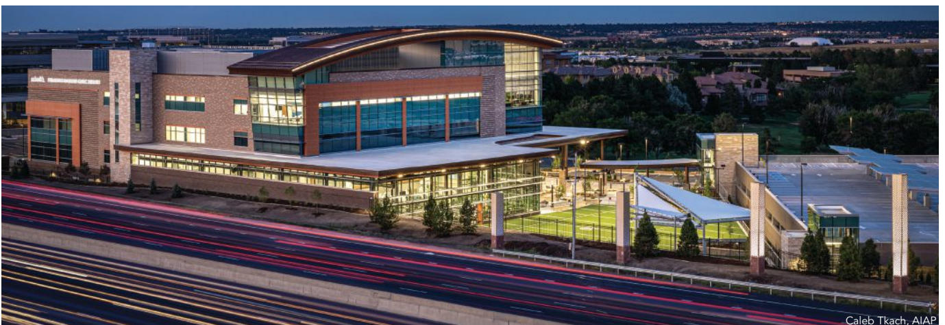
below: The building, including the iconic UCHealth-branded curved roof, is visible from adjacent Interstate 25 in Englewood, Colo.
