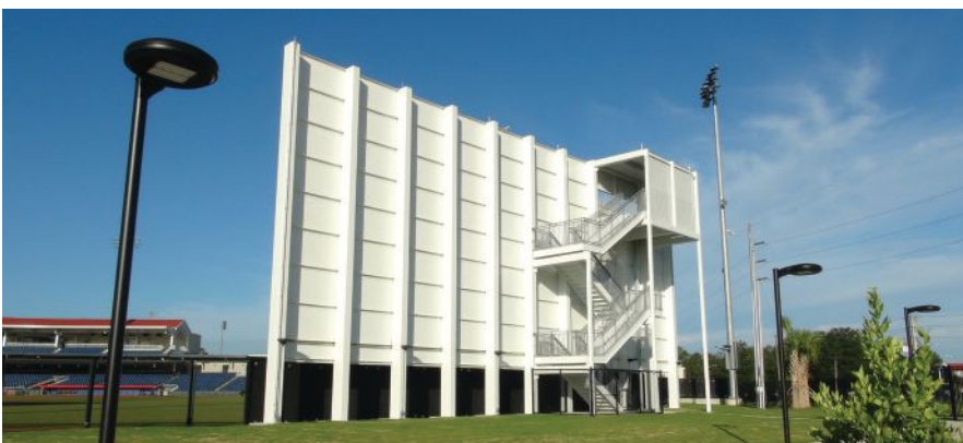
above and below: There was a desire to express as much of the structural steel as possible in all portions of the stadium, including the batter's eye structure in center field, which uses 30 tons of steel.
