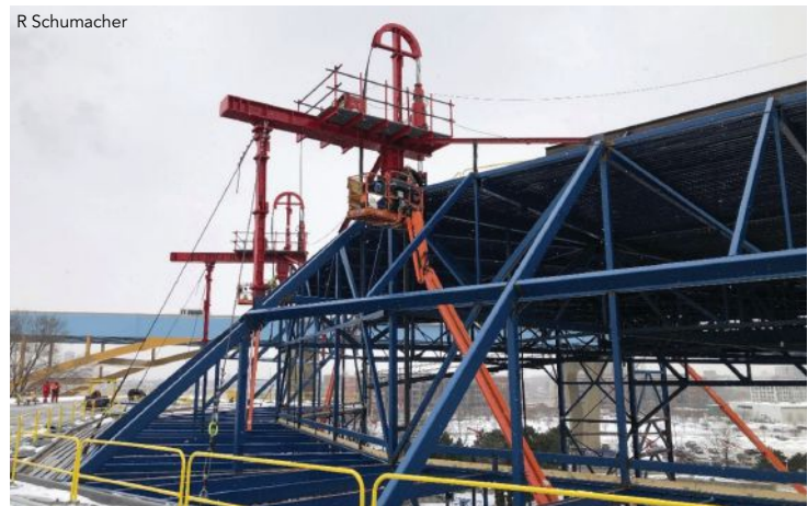
New framing to support the lifted roof.
