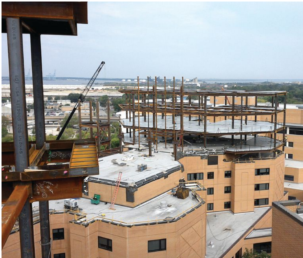
above and below: A change in floor configuration led to a change in framing material, from concrete to steel.
