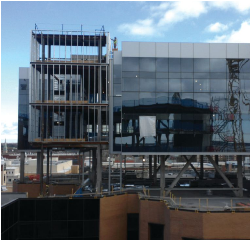
above and below: A change in floor configuration led to a change in framing material, from concrete to steel.
