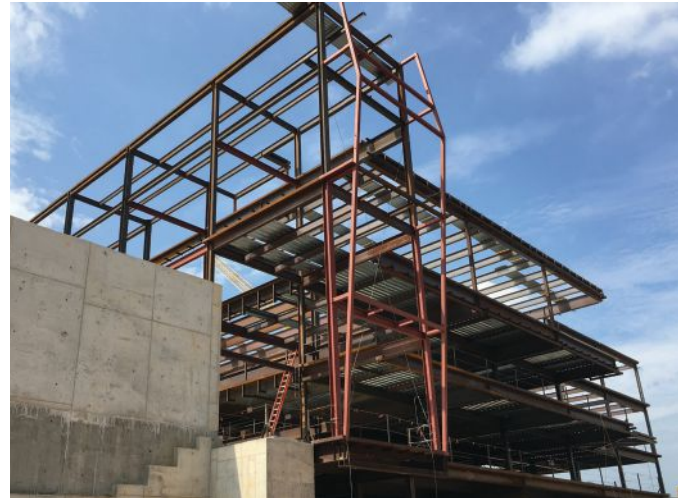
above: An homage to important campus symbols, intersecting groups of arched trusses support the rooftop terrace above the strength training room. The renovated Cole Field House can be seen in the background.
