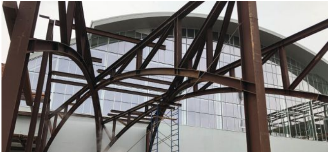
above: An homage to important campus symbols, intersecting groups of arched trusses support the rooftop terrace above the strength training room. The renovated Cole Field House can be seen in the background.
