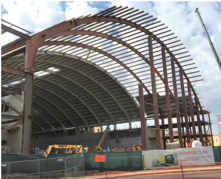
opposite page and above: The bays added to the end of the building were designed to closely match the construction of the existing steel arches that support the roof.
