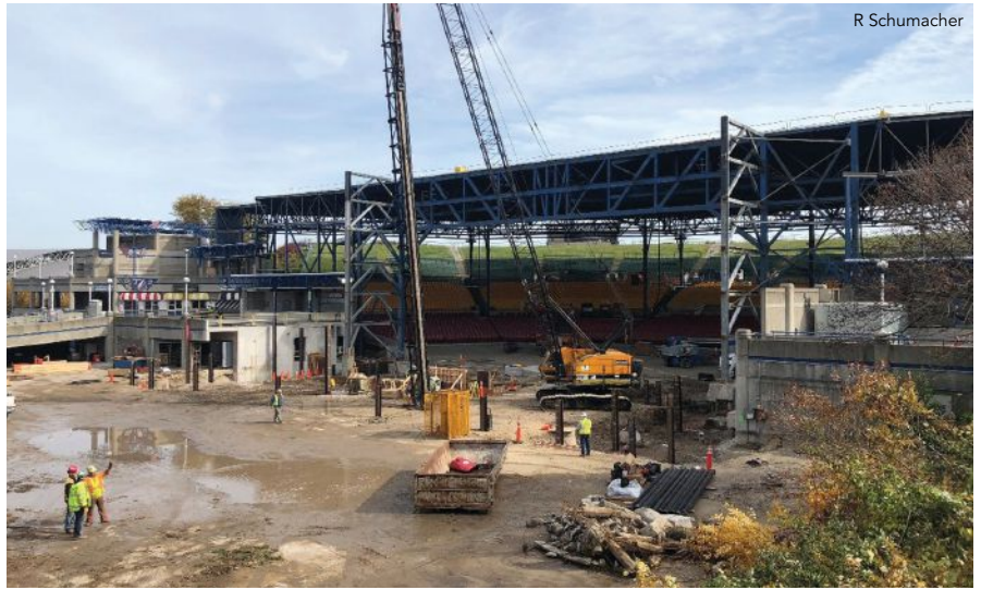
The amphitheater with the stage building demolished and all siding removed.
