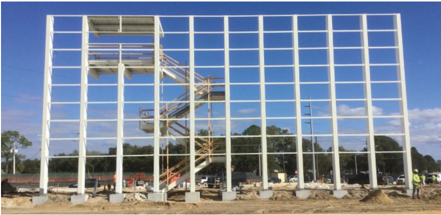
above and below: There was a desire to express as much of the structural steel as possible in all portions of the stadium, including the batter's eye structure in center field, which uses 30 tons of steel.
