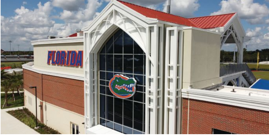
above: The new $55 million, 135,000-sq.-ft stadium can seat 7,000 fans. It was important to the design team that the ballpark tie back to the collegiate gothic style that defines the school's architecture, and steel was the clear choice to accomplish this goal.
