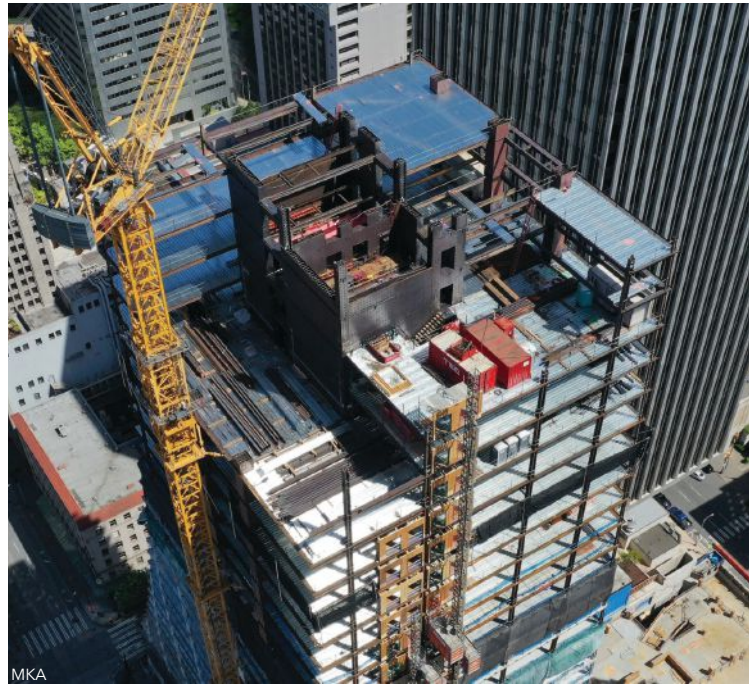
Fig. 2. The Rainier Square project in Seattle, with (left) SpeedCore panels being erected and (right) framing approaching the building's full 850-ft height.
