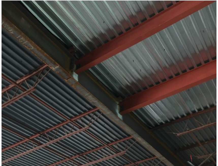
Using structural steel to enhance OWJ framing for added load.
