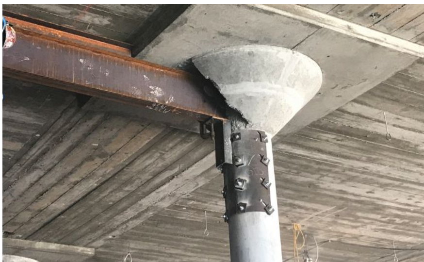
above and below: A floor extension using new steel framing.
