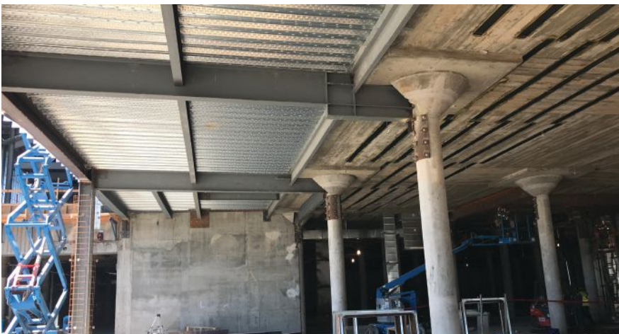
above and below: A floor extension using new steel framing.
