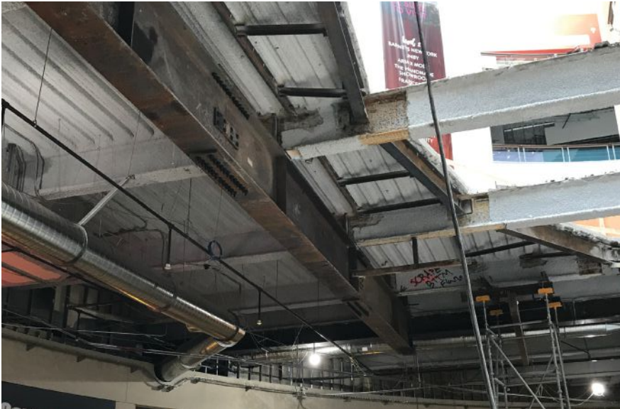
A new underslung beam positioned beneath existing wide-flange steel framing.
