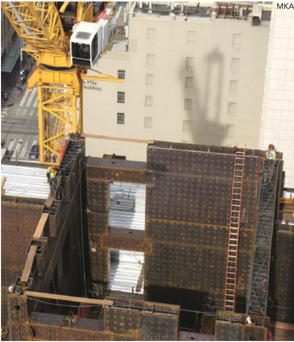
Fig. 2. The Rainier Square project in Seattle, with (left) SpeedCore panels being erected and (right) framing approaching the building's full 850-ft height.
