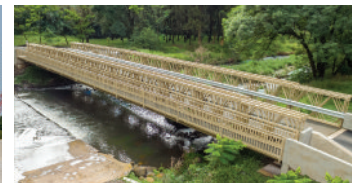
Keahua Garden Bridge - Kauai Island, Hawaii Specified: Duplex (Epoxy & Urethane over Hot Dipped Galvanized)
