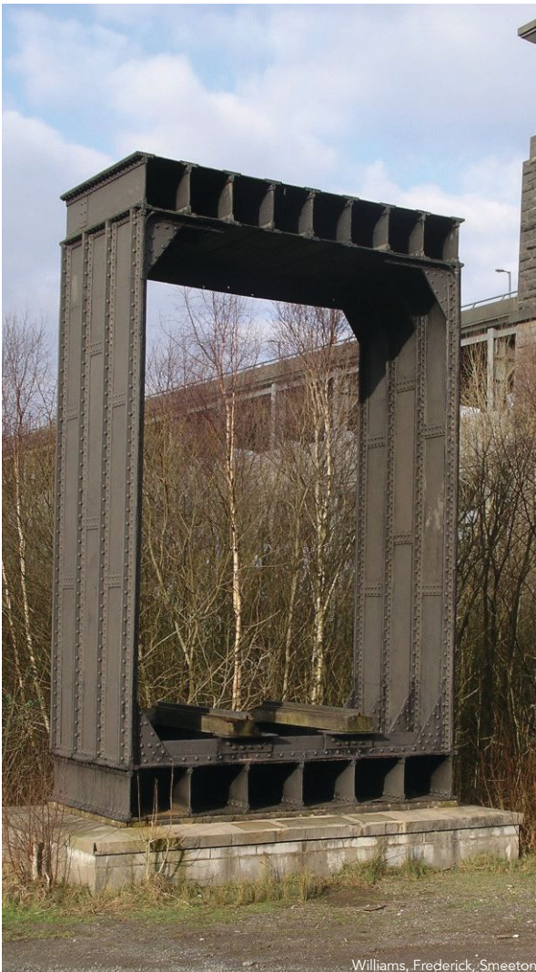
Fig. 3. A section of the original wrought iron tubular Britannia Bridge (left) standing in front of the modern bridge and (right) a rendering of the bridge circa 1852.
