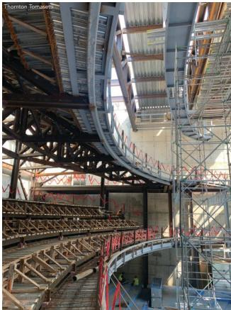
balconies to be constructed while they were supported on temporary columns. During construction, the design team worked with contractor Whiting-Turner, steel fabricator SteelFab, and the steel erector to implement the construction sequence. By coordinating with these parties early on, unwelcome surprises were kept to a minimum and the team achieved the final product as envisioned by HGA.
