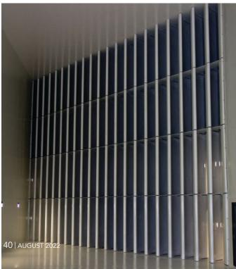
left: The wind tunnel's steel turning vanes, fabricated by Merrill Steel, were successfully installed by Aristeo ironworkers in compliance with the tight customer-required tolerance of  $1_{32}$  in.
