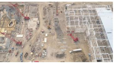
above and below: The majority of the more than 1,800 tons of structural steel was incorporated into the two-story battery lab building and attached support facility, one of the largest steel projects ever for steel fabricator Aristeo.
