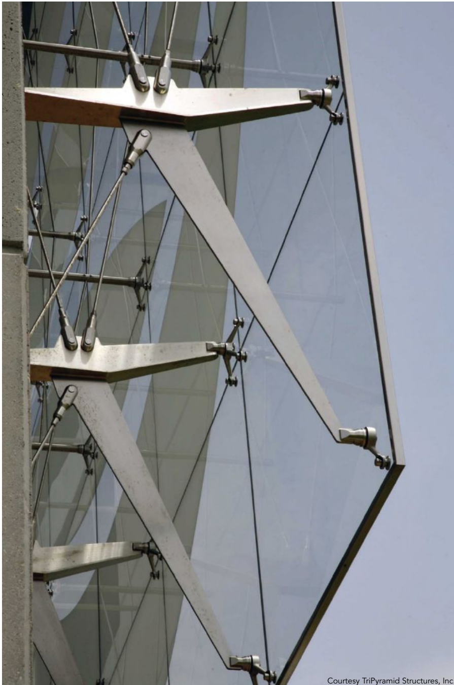
Courtesy TriPyramid Structures, Inc.
