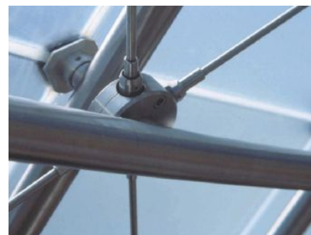
right: This band shell in St. Paul, Minn., was built directly in the flood path of the Mississippi River. The 316L (S31603) structural stainless steel was finished with a very fine grain to reduce the chances of crevice corrosion. The tie rod system is made from cold-drawn stainless steel with a minimum yield strength of 110 ksi.
