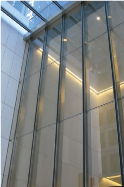
This glass entry in New York City is framed with vertical structural stainless steel mullions. While the design, fabrication, and erection practices needed to execute this type of work are similar to those used for carbon steel, they are not the same. The Stainless Code provides the necessary guidance to properly use these materials.
