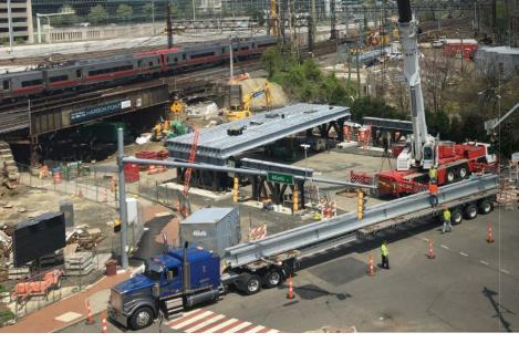
Bridge Stats Span lengths: 70 ft – 70 ft Total structure length: 146 ft  $9^{1}/_{8}$  in. Average structure width: 77 ft 3 in. Steel weight per deck area: 0.16 tons per sq. ft (superstructure), 0.165 tons per sq. ft (total) Total amount of structural steel: 1,785 tons in superstructure, 61 tons in pier plate columns Approximate total cost of bridge: \$48,069,356 Corrosion protection: Hot-dip galvanized
