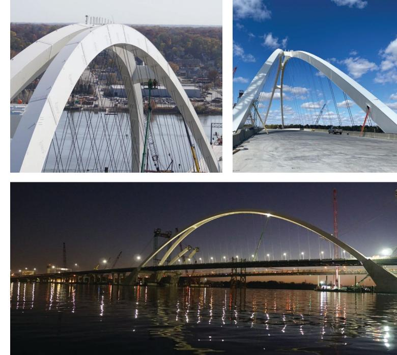
channel as vehicular travelers pass along the corridor between Iowa and Illinois. Because the new steel arch bridge is in a main navigational channel, it took substantial coordination during the construction phase to minimize impacts on river traffic as the arch segments were installed.
