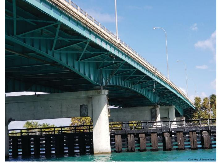
ensure even jacking of the span to avoid racking that could cause deck damage. The FEA model allowed the team to accurately estimate the jacking loads and determine the potential stresses in the top of the deck when a single bearing line was jacked. It also confirmed that jacking the bridge one pier at a time, and not the entire three-span unit at once, was feasible and would not cause unwanted damage.
