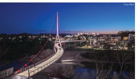
Because of the lightness and slenderness of the bridge deck, it was critical to have horizontal vibration controls. A combination of tuned mass dampers in the bridge transition zones and a pendulum-tuned damper at the main cable termination point created significant damping of the structure.
