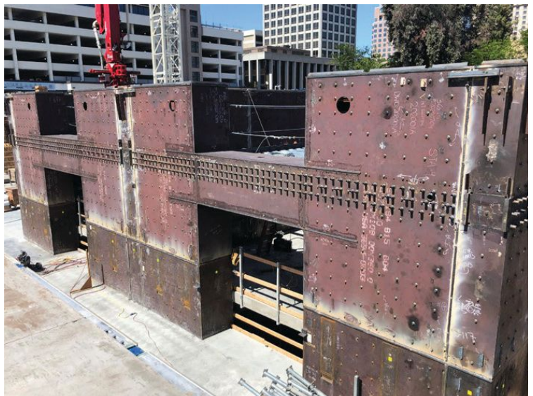
below: Schuff used ½-in. ASTM A572-Gr 55 plate for the vast majority of the core wall elements and required the 1-in.-diameter cross ties to be spaced at 12 in. center-to-center in the lower regions of the building before transitioning to 18 in. center-to-center for the upper floors.
