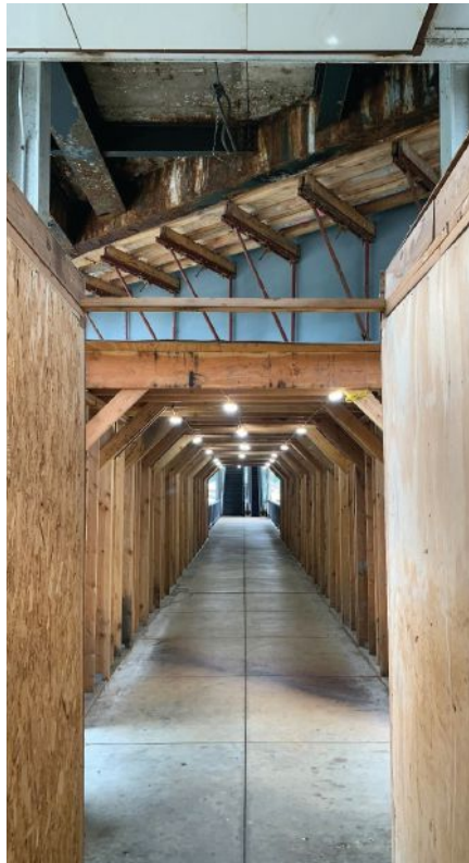
A temporary shield was put in place to protect CTA riders crossing under the bridge during construction.
