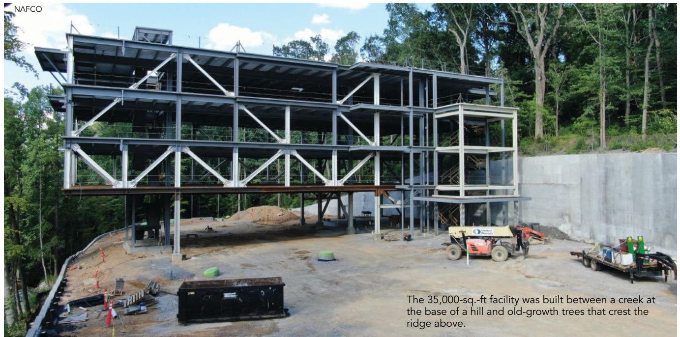
The building employs a floor-to-floor truss system that eliminates interior columns and allows for abundant light to flood in through the prominent glass that joins with metal panels to wrap the building in both metal and light.
