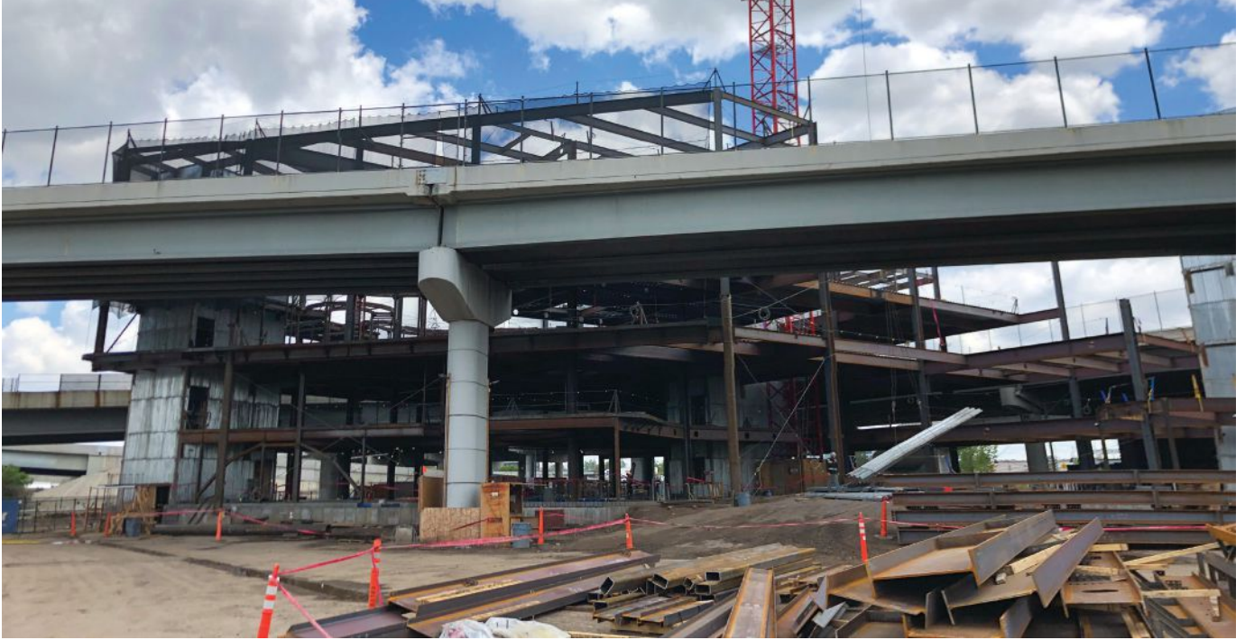
above: The steel had to be hauled underneath an overpass from its laydown area before it could be hoisted by crane.
