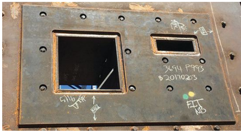
below: Openings in the panels for routing MEP systems.
