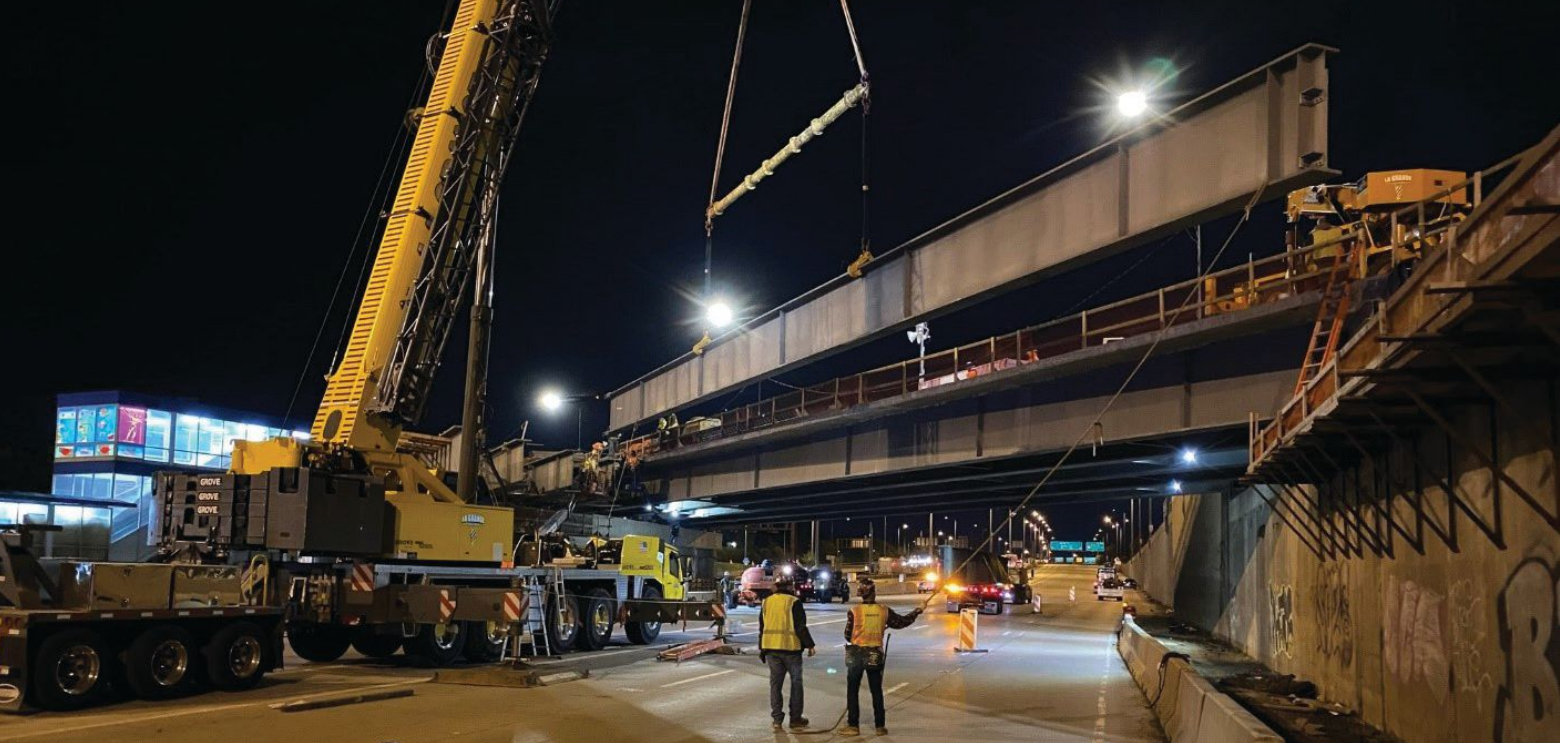
Erecting the Span 3 girder over I-90/94.
