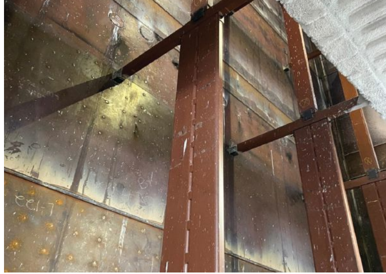
above: Bracing in an elevator core.
