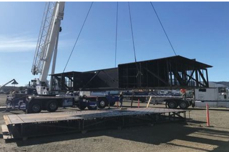
Hoisting a SpeedCore panel onto a truck.
