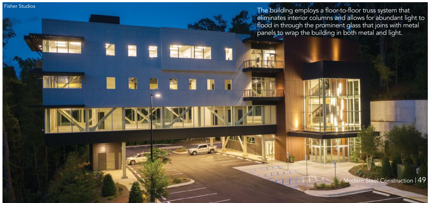
The 35,000-sq.-ft facility was built between a creek at the base of a hill and old-growth trees that crest the ridge above.
