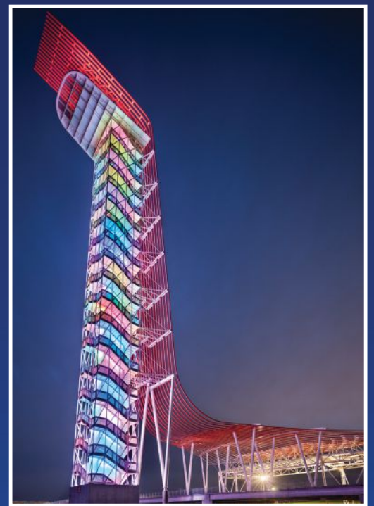
2015 IDEAS 2 Merit Award - 73 pieces of curved 8" sch 40 pipe totaling 35 tons for Circuit of the America Observation Tower. Austin, TX
