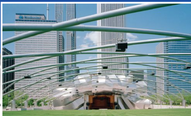
2005 EAE Merit Award - 570 tons of 12", 14", 16", 18" and 20" pipe curved for the Jay Pritzker Pavilion. Chicago, IL
