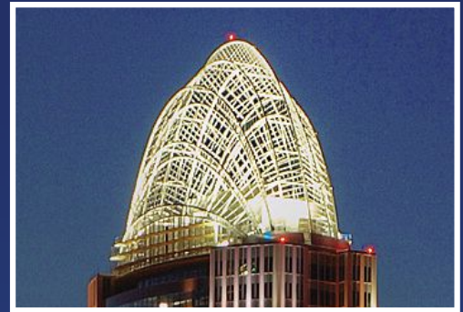
2012 IDEAS 2 Merit Award - 133 tons of 16" pipe curved for the Rooftop Tiara of the Great American Tower at Queen City Square. Cincinnati, OH
