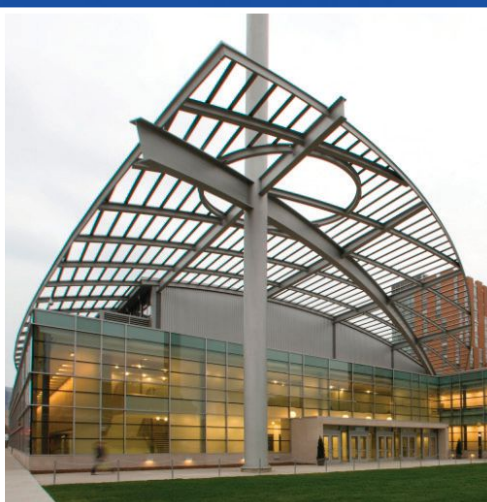
2010 NCSEA Award Winner - 200 tons of beams, channels and angle for the roof of the University of Illinois at Chicago Forum. Chicago, IL
