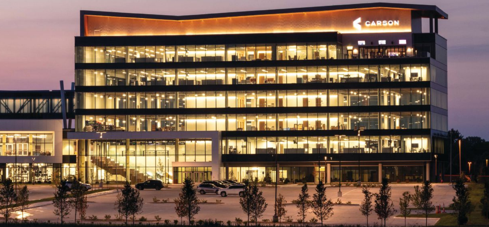
The new Carson headquarters building is part of the 500-acre Heartwood Preserve development located in Omaha.
