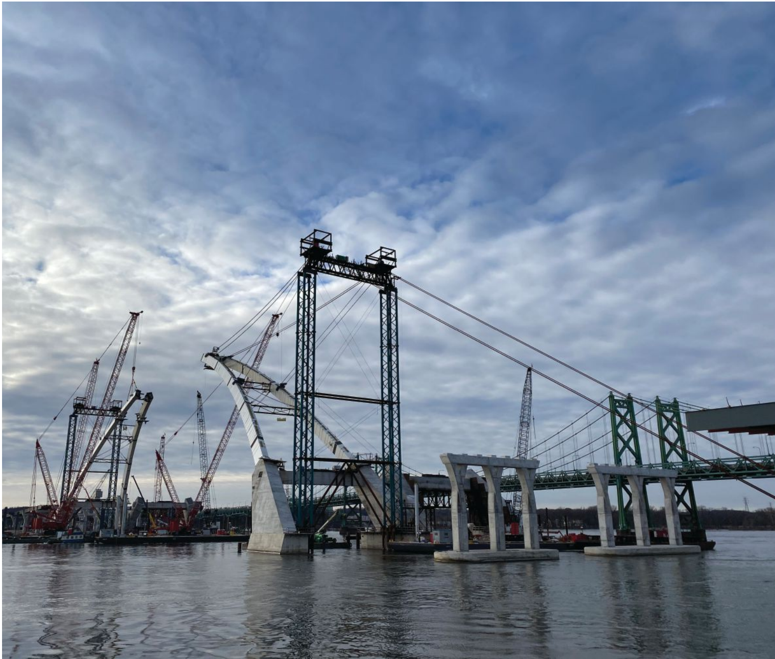
above: A view of the westbound bridge arch with 20 of the 30 arch segments installed.
