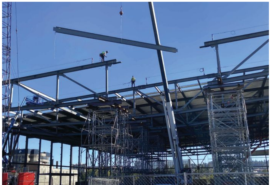
above and below: Erecting the trusses. To speed up erection, full-penetration welds were all performed in the shop, and truss chord splice connections and truss web end connections were bolted in the field.
