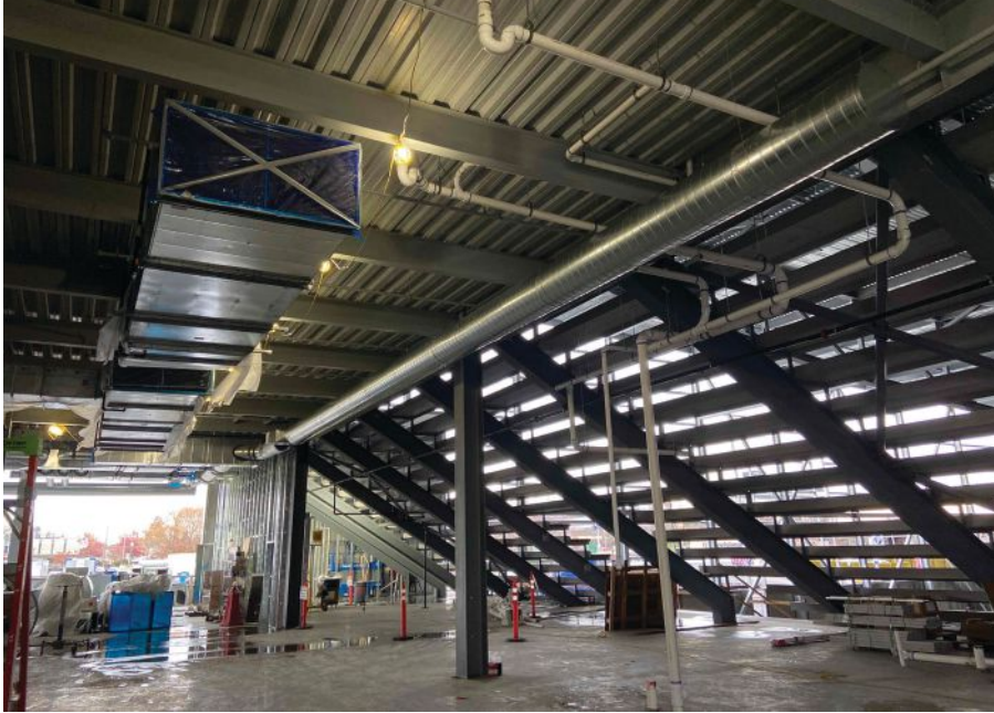
above: Steel stringer bracing for the bleachers.
