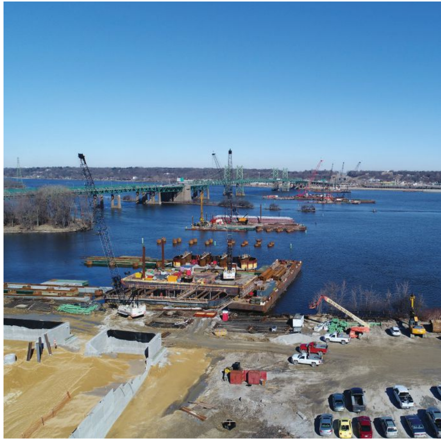
below: Erecting a steel arch segment on the Iowa side of the river.
