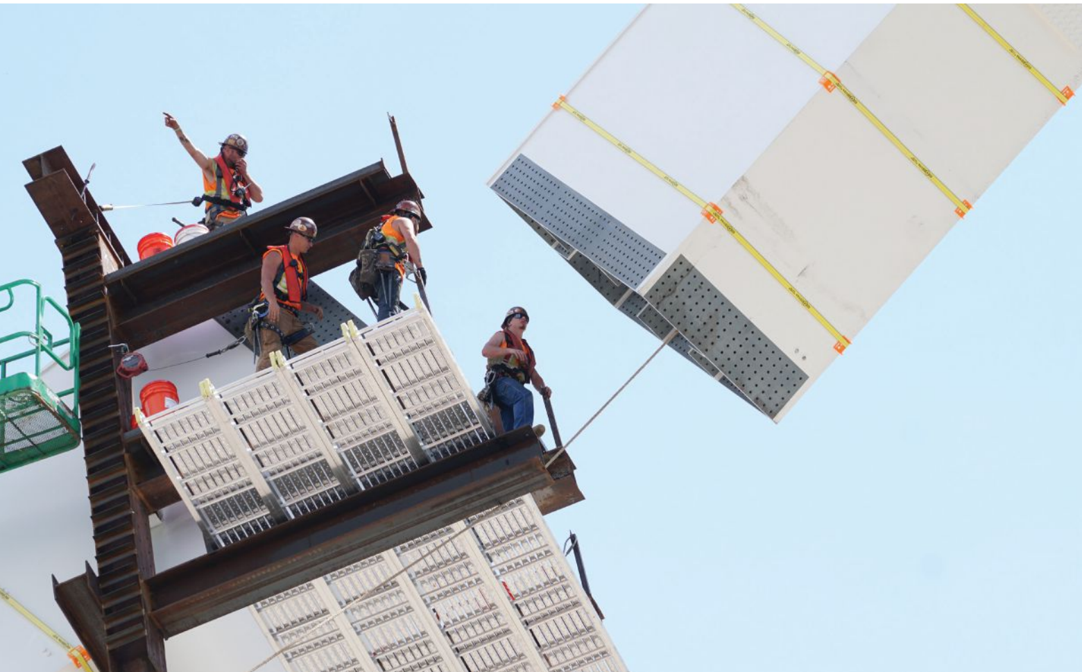
below: Erecting a steel arch segment on the Iowa side of the river.
