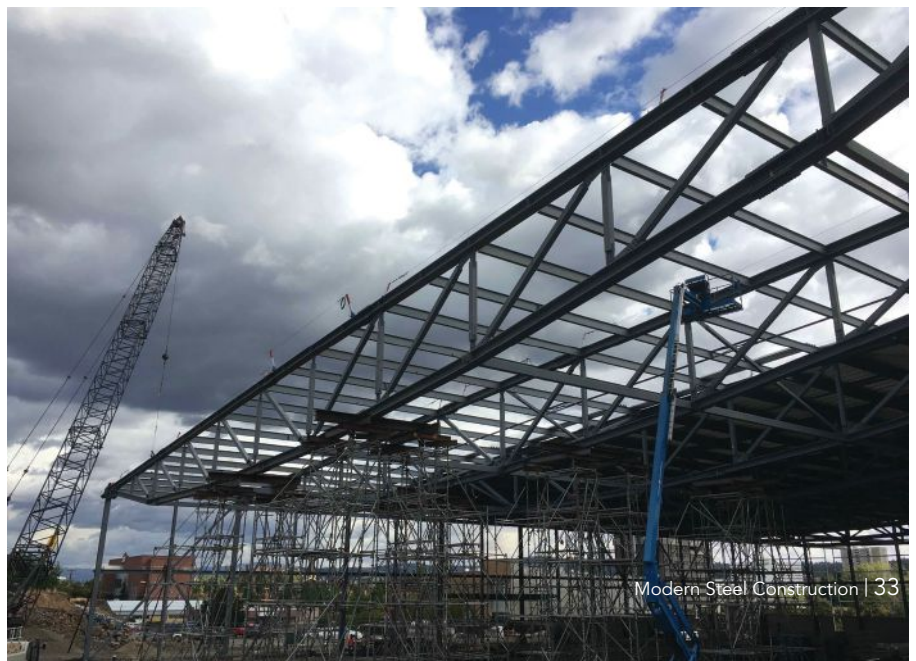
above and below: Erecting the trusses. To speed up erection, full-penetration welds were all performed in the shop, and truss chord splice connections and truss web end connections were bolted in the field.
