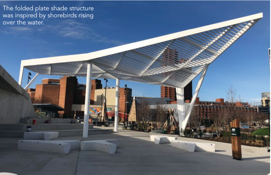
The completed roof structure is 32 ft wide and 80 ft long.
