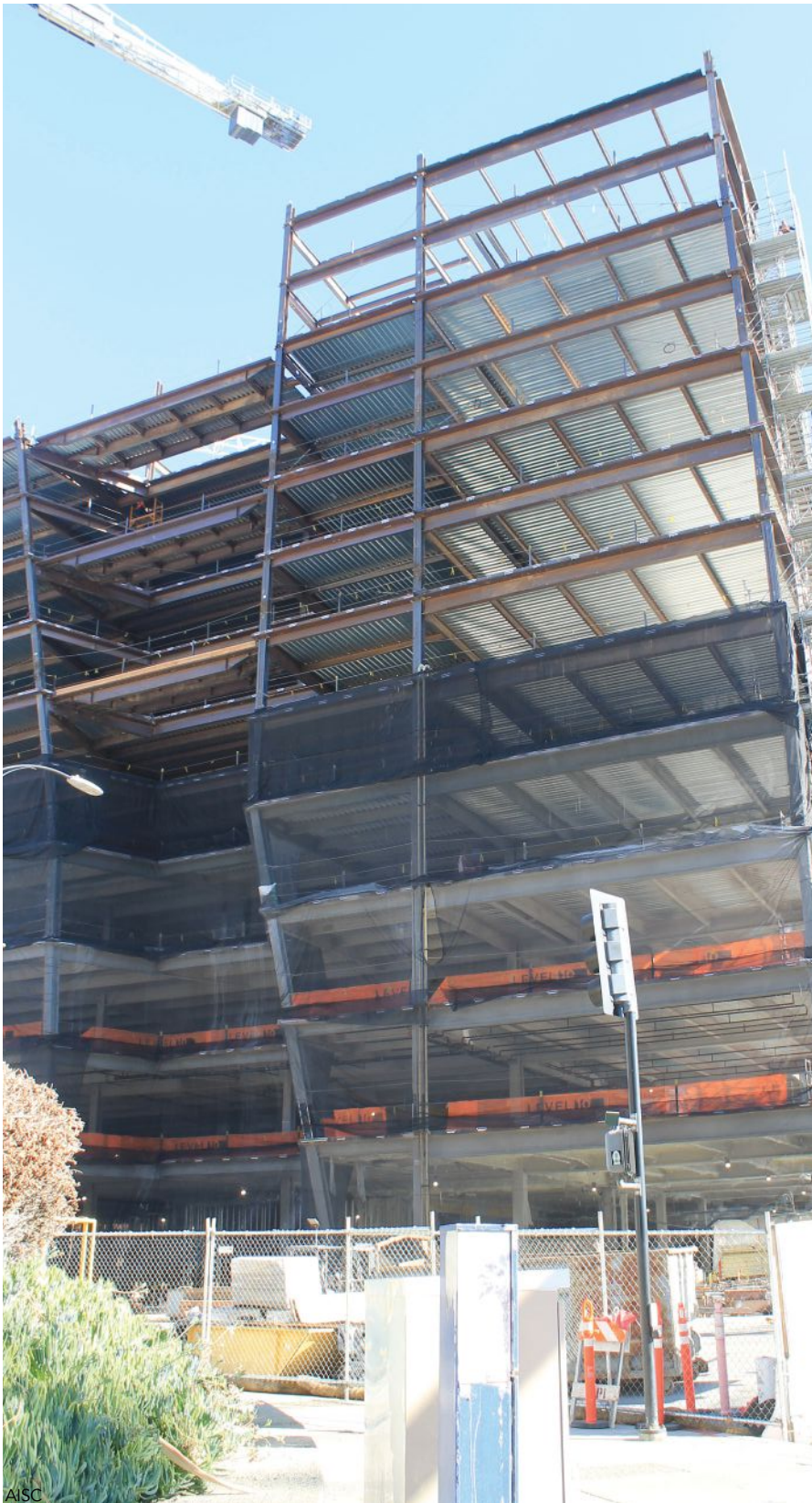
Fig. 6. 200 Park in San Jose, also designed by MKA, is the second building to implement the SpeedCore system.
