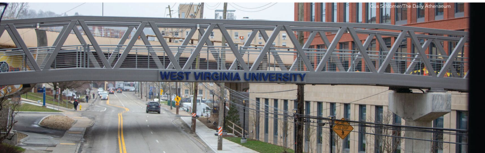
above and below: The architectural design of the pedestrian bridge mandated an "open-to-the-sky" approach with no cross-bracing members between the panel points of the truss top chords.
