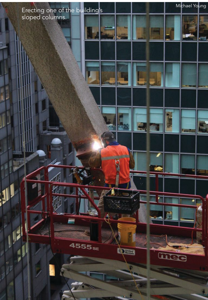
Solid steel nodes located at the transitions between regular and sloped columns were sculpted to match the shape of the sloping façade.
