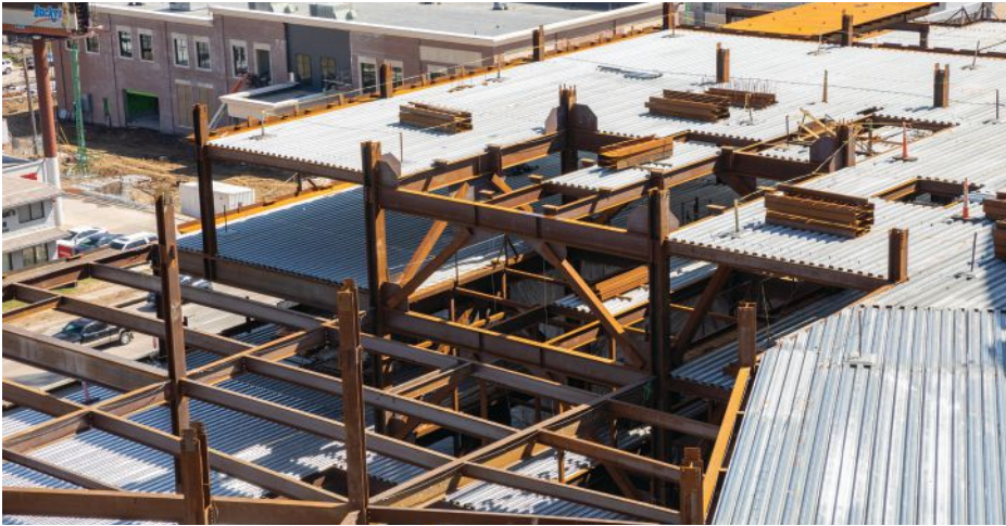
above and below: In all, the project incorporated 3,569 tons of steel. Typical bay sizes are 32 ft by 32 ft, and typical columns are W14 sections, with the largest being a W14x730 located at a couple of braced frame locations.
