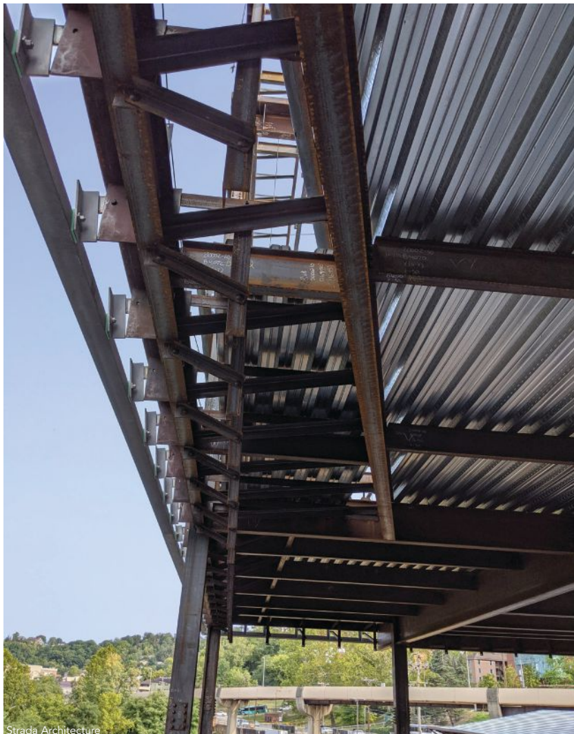
below: The project incorporated 145 tons of steel for façade support.
