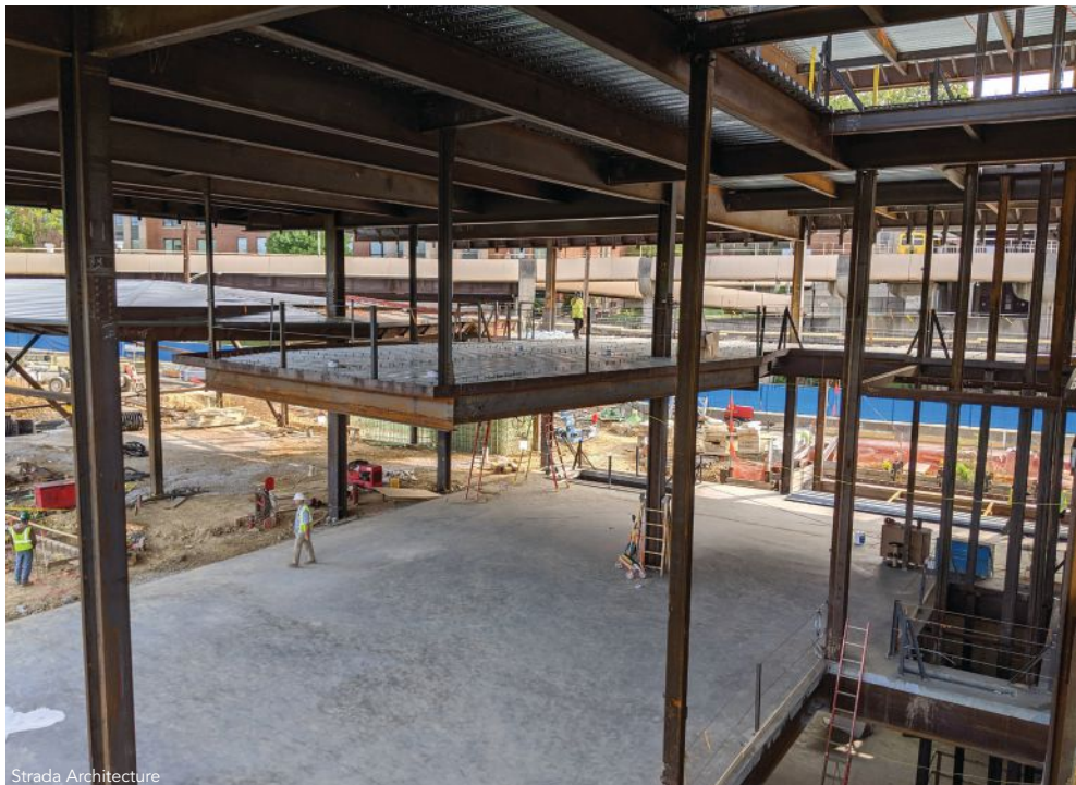
In order to make the Ideation Hub (framing above, completed below) appear to float, this element was framed using three strategically located hangers and four cantilevered beams.
