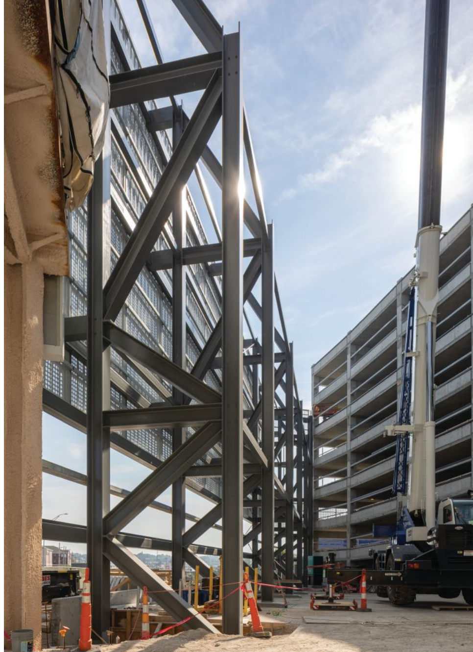
above and below: The building's signature screen wall is built with 10-ft-deep braced frames spaced at 28 ft and tied together with structural steel to brace them out-of-plane.
