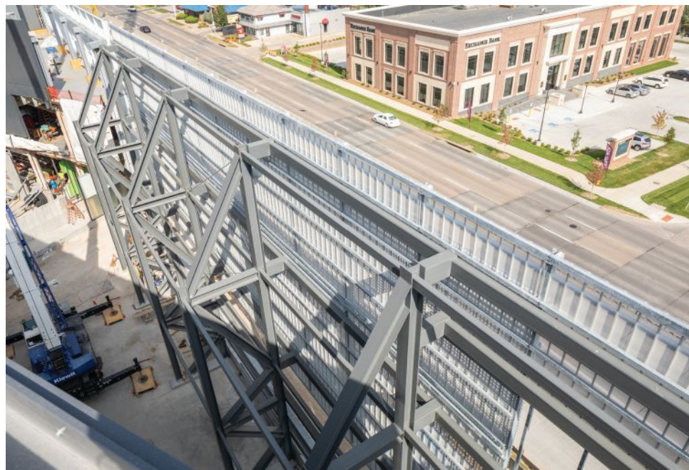
above and below: The building's signature screen wall is built with 10-ft-deep braced frames spaced at 28 ft and tied together with structural steel to brace them out-of-plane.
