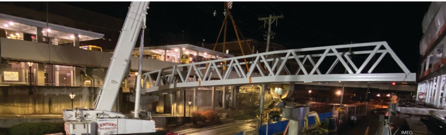
above and below: The architectural design of the pedestrian bridge mandated an "open-to-the-sky" approach with no cross-bracing members between the panel points of the truss top chords.
