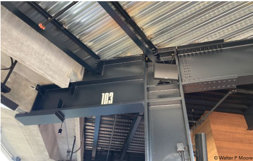
above and below: Another look at steel supporting the seating. The entire structure uses 6,000 tons of steel in all.
