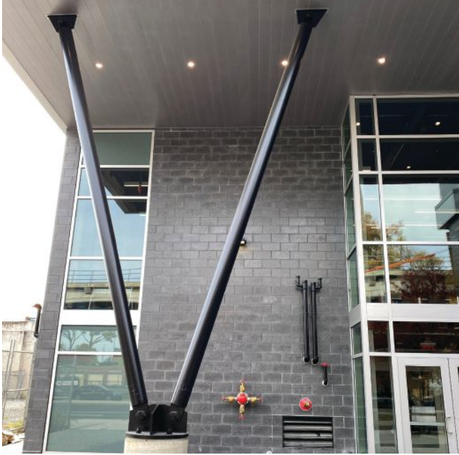
One unique aspect of the steel framework is the two-story V-shaped column supporting a canopy roof over the north entrance to the building.
