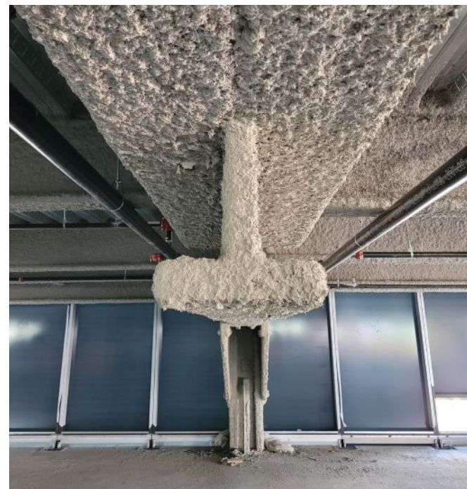
above and below: Two views of the cut-out portion of the transfer truss, which was designed to alleviate a low head height condition without having to adjust the floor-to-floor height at the level under the transfer truss.
