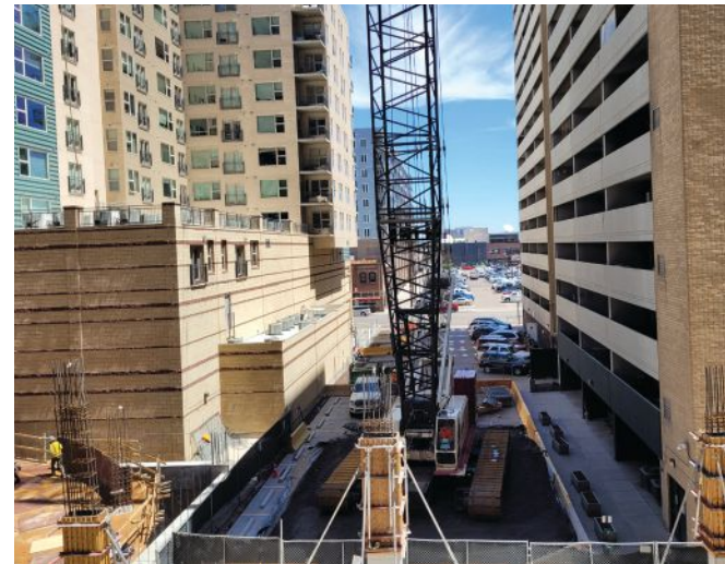
below: The construction team took advantage of an empty street adjacent to the project for crane staging and material delivery and laydown.
