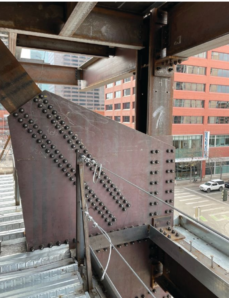
below: The actual bolted connections.
