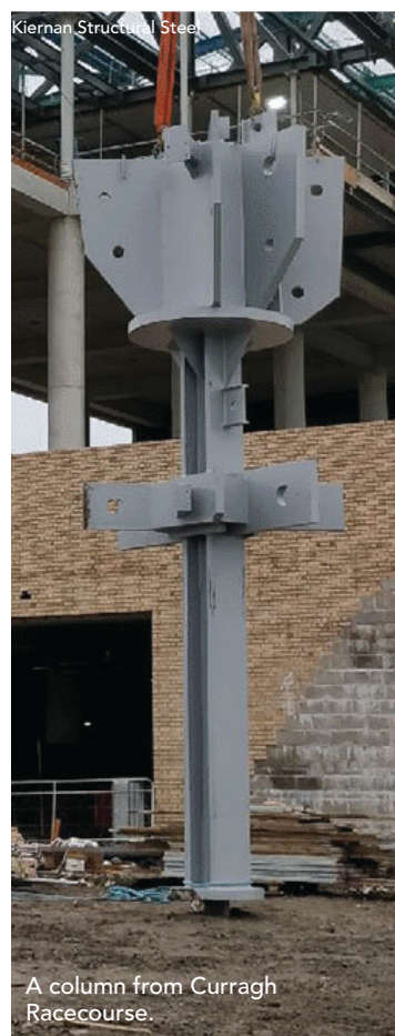
A column being fabricated for use at Curragh.
