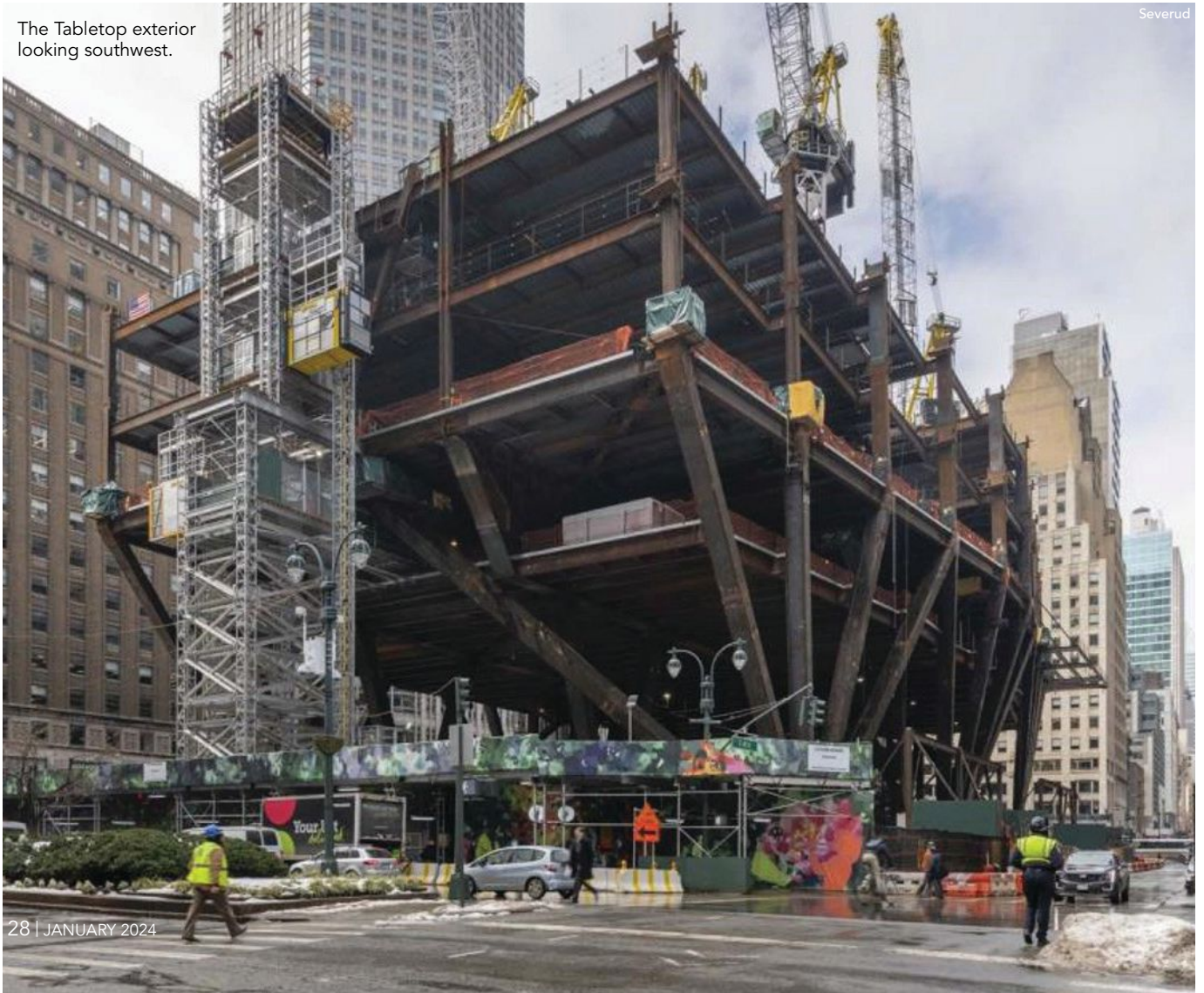
Subway tracks below the building site necessitated a two-story-high arrangement of steel transfer girders called the Tabletop.
