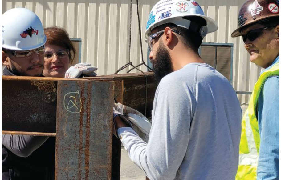
above: UT-Tyler students get hands-on experience erecting steel.
