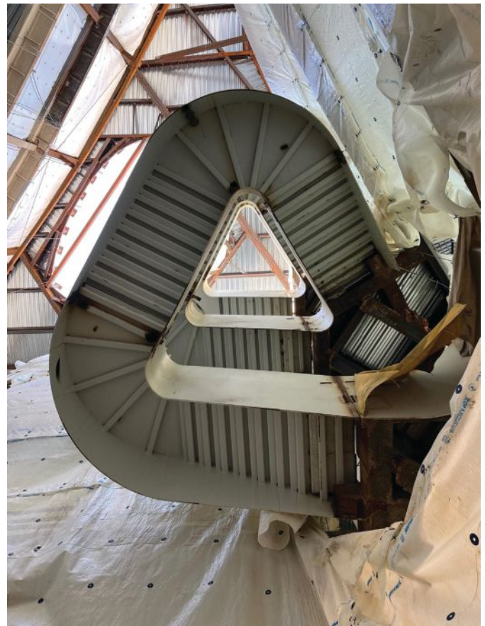
below: Looking upward from directly below the stair.
