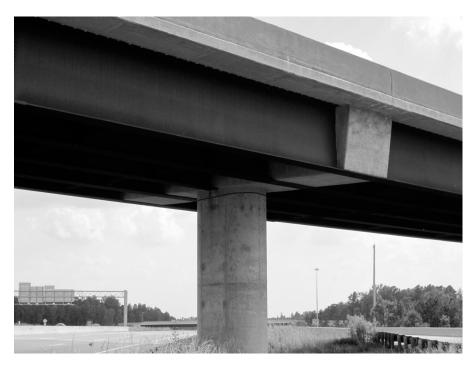
Figure 3.15.1-6. An integral post-tensioned concrete pier cap used in an interchange in Raleigh, NC to avoid a conventional concrete rectangular cap (concrete drop cap). This allows the use of a radial cap while still maintaining adequate vertical clearances over traffic below the bridge.
