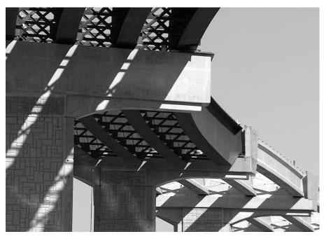
Figure 3.15.1-7. Dapped ends on curved steel plate girders resting on an inverted-tee bent cap on a bridge in Texas. In this case, the dapped girder ends were used to match the depth of the precast girders in the next span; but this same concept could be used to allow use of a radial bent cap the same depth as the girders, providing an effect similar to that of an integral bent cap.
