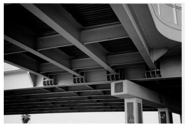
Figure 4.7.5-1. Framing of an elevated T-intersection steel girder bridge in McAllen, Texas. The intersecting span is supported on a series of steel corbels formed of partial-depth stiffeners with a cap plate.
