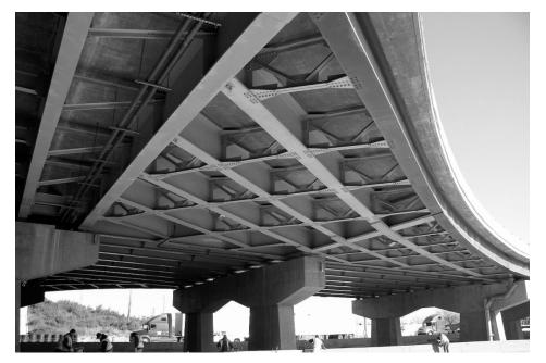
Figure 4.7.6-2. View of curved infill-framing area between two orthogonal regions of conventional parallel stringer framing in one of the ramp flare areas of an SPUI bridge structure.
