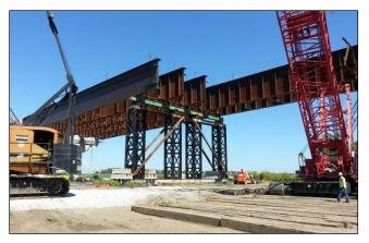
Figure 5: Temporary Bents Utilized During Girder Erection of the Main Steel Unit
