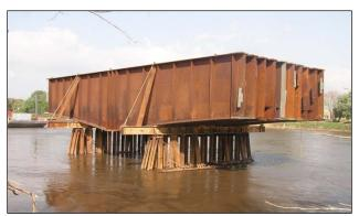
Figure 4: Storage of Haunched Steel Girder Pier Segments on Custom Built Racks in River
