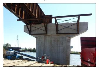
Figure 6: Temporary "Wing" Struts for Interior Pier Steel Section Support During Erection
