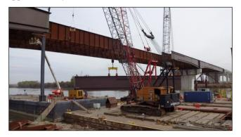
Figure 7: Erection of Drop-In Steel Segments at Main Span
