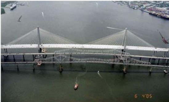
(a) Aerial view
