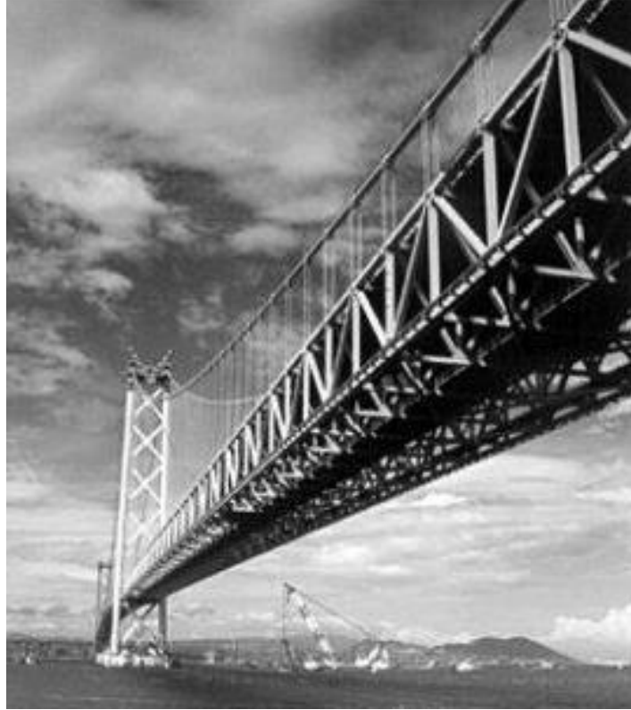
Figure 33. Akashi Kaikyo Bridge, longest suspension span (6530 ft) (courtesy of www.structurae.de ).
