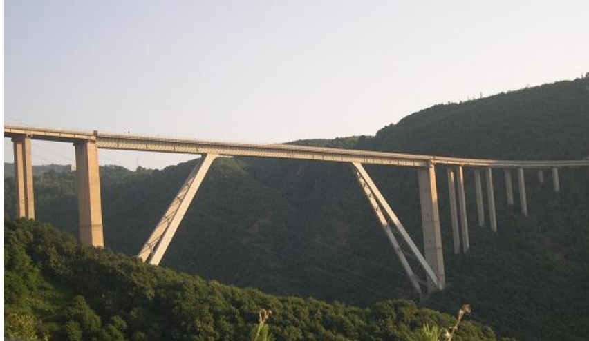
Figure 25. Sfalassà Viaduct in Calabria, Italy, longest box-girder span, 1230 ft (courtesy of www.structurae.de ).
