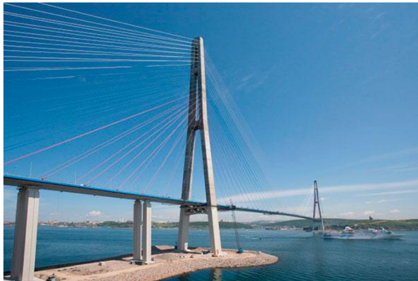
Figure 34. Russky Island Bridge, longest cable-stayed span in the world (3260 ft) (courtesy of Road Traffic Technology).
