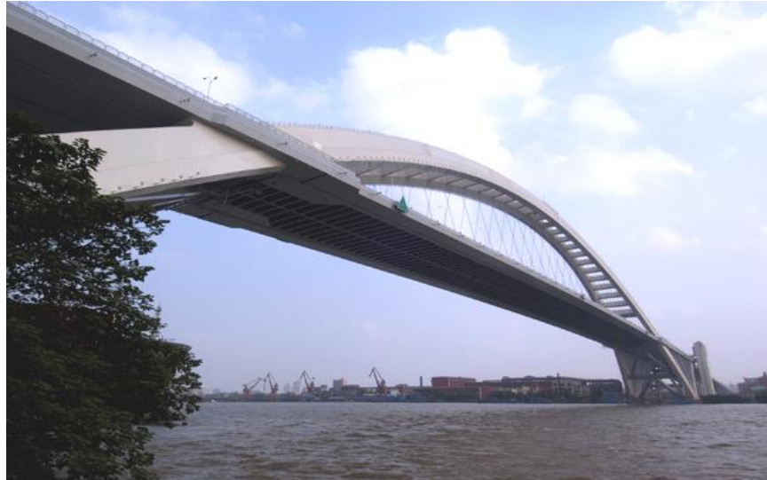
Figure 30. LuPu Bridge deck system (courtesy of www.structurae.de ).
