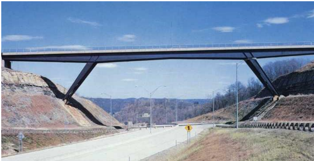
Figure 28. Slant-legged rigid-frame bridge (courtesy of HDR).
