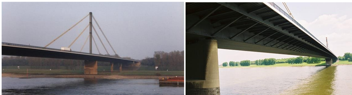
(a) Overall view
