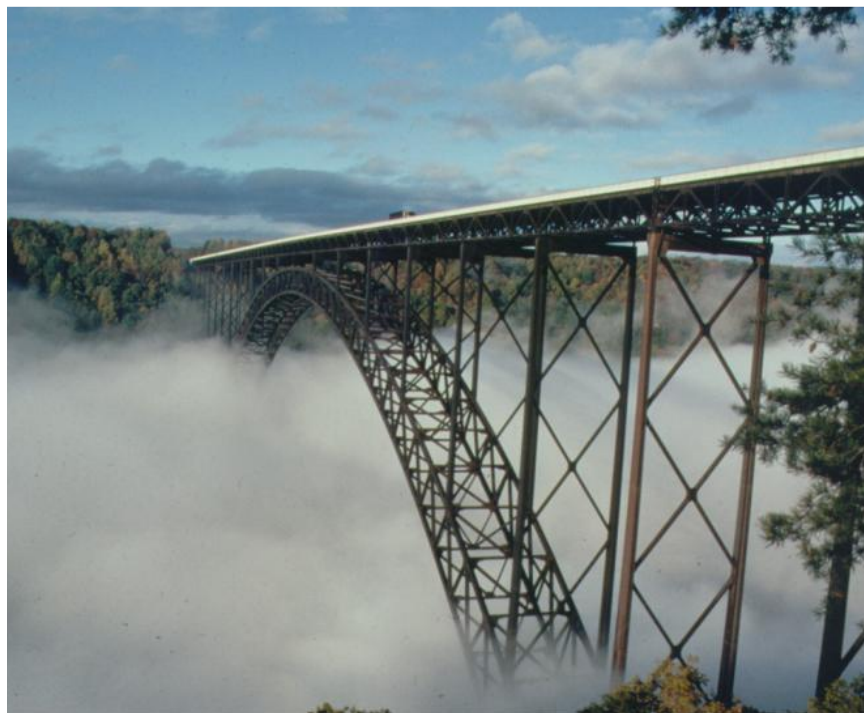
Figure 31. New River Gorge Bridge in West Virginia, longest span steel arch in the United States, 1700 ft (courtesy of HDR).
