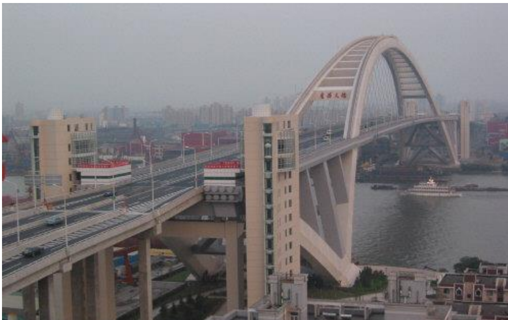
Figure 29. LuPu Bridge in Shanghai, China, longest span steel arch, 1800 ft (courtesy of www.structurae.de ).
