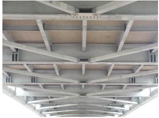
Figure 9 Photo of a typical framed floor system
