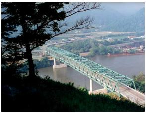
Figure 6 Photo of a steel through truss bridge (Chelyan Bridge over Kanawha River, Kanawha County, West Virginia) (Note the top chord lateral bracing and the portal bracing)
