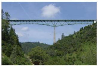
Figure 5 Photo of steel deck truss bridge (Foresthill Bridge over American River's North Fork, Auburn, California)
