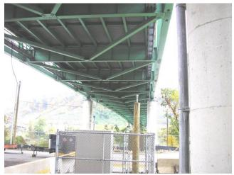
Figure 8 Photo showing a typical stacked floor system
