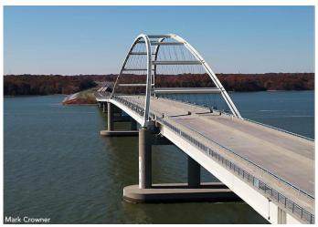
Figure 11 Photo of a steel tied arch bridge (Kentucky Lake Bridge in western Kentucky)
