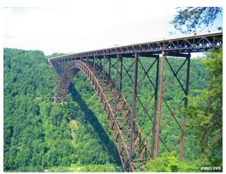
Figure 10 Photo a steel deck arch bridge (New River Gorge Bridge near Fayetteville, West Virginia)
