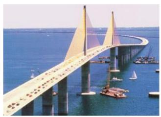
Figure 15 Photo of a cable-stayed bridge with single column towers (Sunshine Skyway Bridge, Tampa Bay, Florida)
