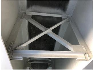
Figure 1 Photo of a typical multi-girder system with x-type intermediate cross-frames
