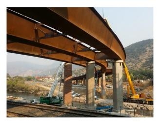
Figure 3 Photo of a typical tub girder bridge under construction (Credit: RS&H)
