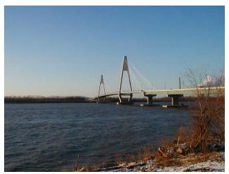
Figure 13 Photo of a cable-stayed bridge with A-Towers (William H. Natcher Bridge over Ohio River near Owensboro, Kentucky)
