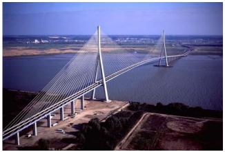
Figure 14 Photo of a cable-stayed bridge with inverted Y-Towers (Normandy Bridge over Seine River near Le Havre, France)
