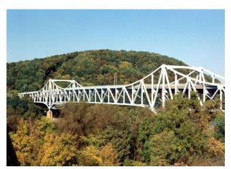
Figure 7 Photo of a steel half-through truss bridge (Glenwood Bridge over Monongahela River, Pittsburgh, Pennsylvania)
