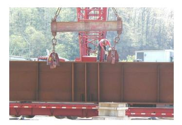
Figure 9 Use of a spreader beam for I-girder erection
