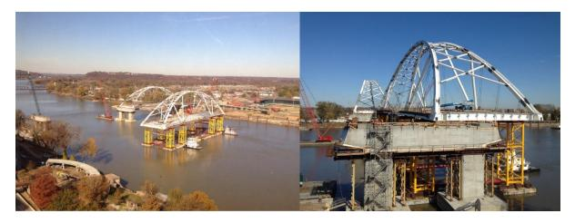
Figure 19 Tied arch sliding laterally in place, by use of barges
