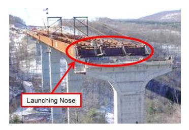
Figure 12 I-girder launch with launching nose and cable tie-backs
