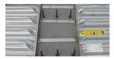
Figure 20 SIP forms attached to a top flange in a tension region
