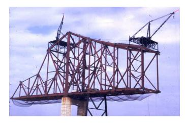
Figure 14 Cantilever erection of a continuous truss using derricks
