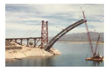
Figure 15 Arch erection using stay towers and cables
