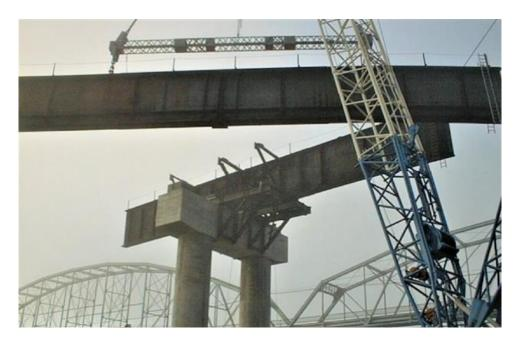
Figure 8 Pier brackets in an I-girder bridge
