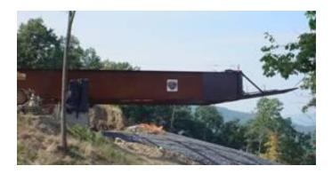
Figure 11 I-girder bridge launching
