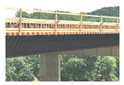
Figure 21 Typical overhang brackets
