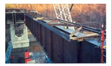
Figure 25 Temporary top flange stiffening truss
