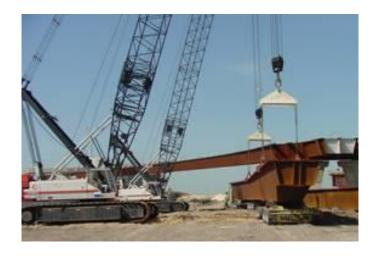
Figure 10 Box girder erection using two crawler cranes
