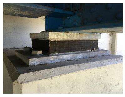
Figure 1 Elastomeric Bearing (courtesy R. J. Watson)
