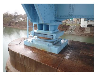
Figure 2 Pot Bearing (courtesy HDR)
