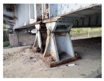
Figure 4 Fixed Mechanical Bearing (courtesy HDR)
