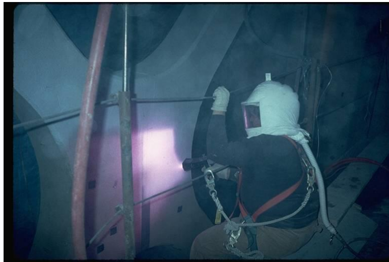
Figure 5. Photo. Metalizing of a bridge member in the field (photo courtesy of R. Kogler).
