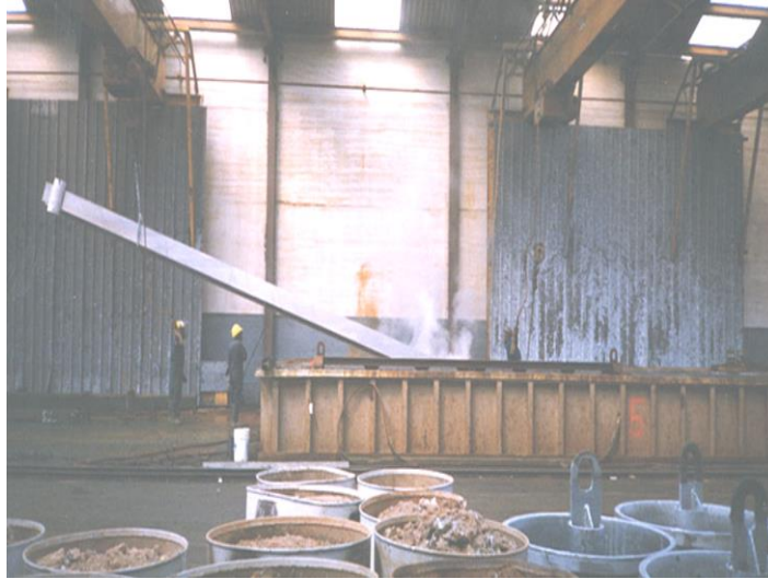
Figure 7. Photo. Hot dip galvanizing kettle with long beam being dipped at one end.
