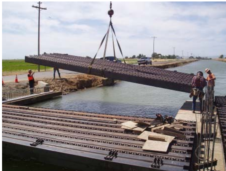
Photo courtesy of Mittal Steel
