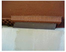
Figure 23: The simplicity of steel-reinforced neoprene bearings illustrated in an expansion bearing at the end of an 880-foot continuous tub girder unit
