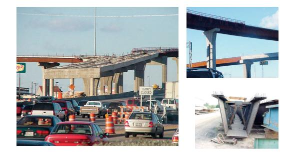
diaphragms and fewer girders versus plate girder alternates can speed erection, a critical advantage in urban highway reconstruction projects where traffic interruptions (and associated contractor "lane rental" penalties) dramatically affect construction costs and pose economic impacts to the community.
