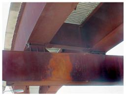
Figure 16: At supports, full-depth plate girder sections are often used for external diaphragms.
