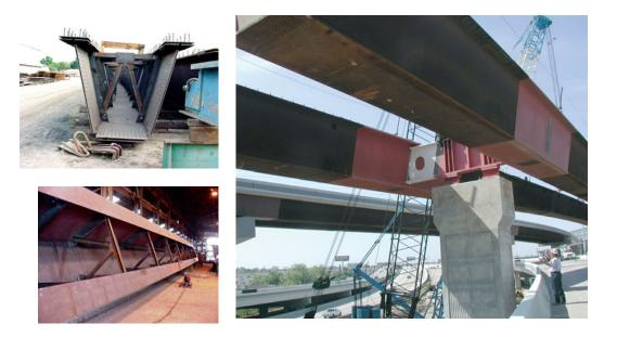
The effects of transverse loading on the weld because of web slope and lateral bracing loads should be included...
