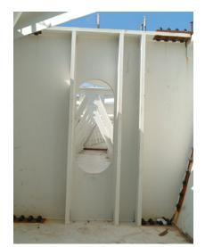
Figure 13: Internal diaphragms at supports generally use full-depth solid webs, with access manholes between the bearing stiffeners.
