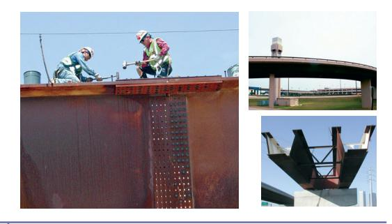
(in excess of 14 feet) can outweigh costs of adding additional field splices. In rare cases, tub girders are so wide they must have longitudinal field splices in bottom flanges.
