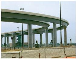
Figure 2: Steel tub girders under construction for a new Automated People Mover system. Tight curvature and clean appearance were key factors in choosing steel tub girders.
