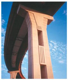
Figure 1: A bold statement in modern highway bridge design, steel tub girders offer advantages in span range, ability to accommodate curvature, and aesthetics.
