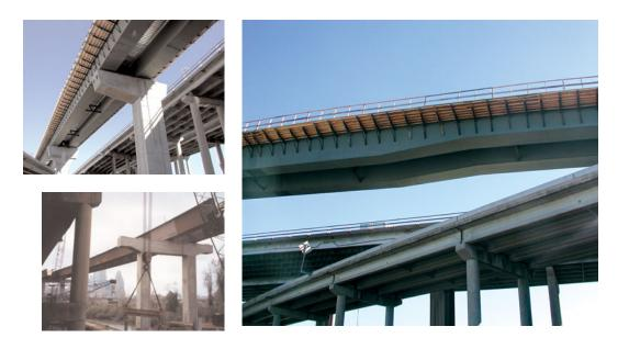
Designers should also realize that in many cases, there are no hard and fast rules associated with these issues... Steel tub girders are often an excellent choice for modern highway bridge superstructures. They offer advantages over other superstructure types in terms of span range, stiffness, and durability – particularly in curved bridge applications. In addition, steel tub girders have distinct aesthetic advantages, due to their clean, simple appearance.
