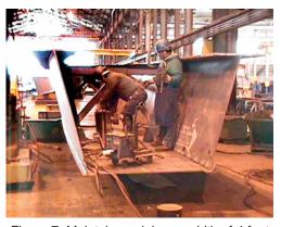
Figure 7: Maintain a minimum width of 4 feet for tub girders to allow room for workers to complete fabrication of various internal details.
