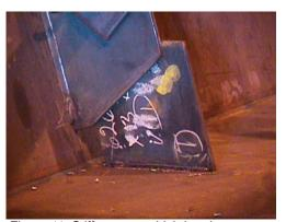
Figure 11: Stiffeners to which bracing members are attached should be connected to girder flanges to reduce local distortion. Shown is a typical detail for connection to the bottom flange.
