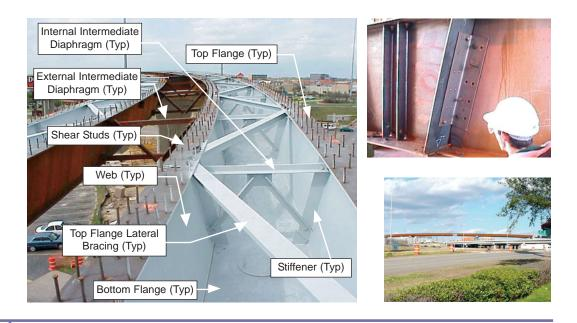
The girder design process for tub girders should begin with development of a framing plan. Many decisions made early in the design process can have significant impacts later on; some basic issues are presented below. Structural analysis as discussed above must be performed to derive the load effects, which are subsequently checked with the code provisions.
