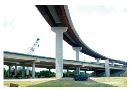
Figure 5: Simple lines, smooth surfaces, and fewer parts visible; the clean appearance of tub girders offers distinct aesthetic advantages.
