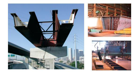
utilize a K-frame configuration, with depth closely matching girder depth for efficiency and simplification of supporting details.
