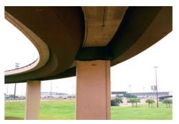
Figure 4: Steel tub girders built on horizontal radii as tight as 175 feet were constructed at the Dallas/Fort Worth International Airport in the late 1970s.
