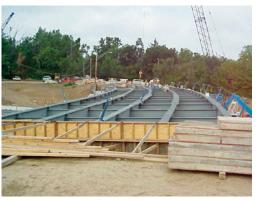
Figure 3: For slight curvature and spans below approximately 120 feet, other superstructure types, such as the curved steel plate girders in this shallow depth curved grade separation bridge, may be a better choice than steel tub girders.
