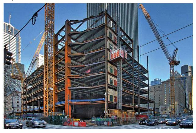
Steel erector for the 850-ft-tall Rainier Square Tower, which has a radical new composite steel superstructure, says construction is proceeding at a rate of 1.36 floors per week.
